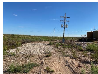
Photograph 14: Northern view of the pasture release extent.
