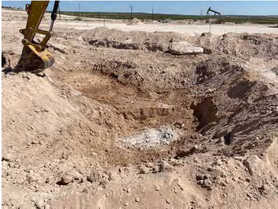
Photograph 3: South facing view during excavation activities.
