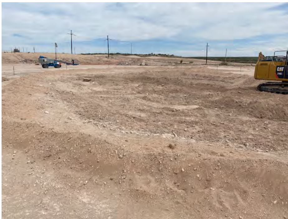
Photograph 2: East facing view during excavation activities.
