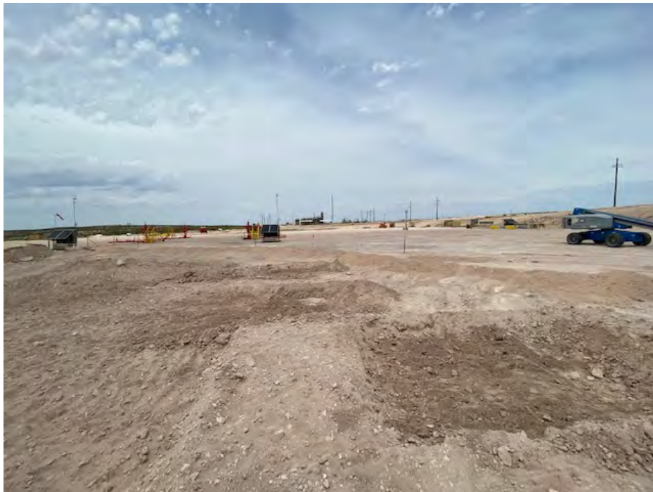
Photograph 4: North facing view during excavation activities.
