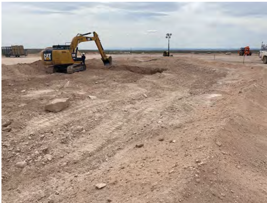
Photograph 1: West facing view during excavation activities.
