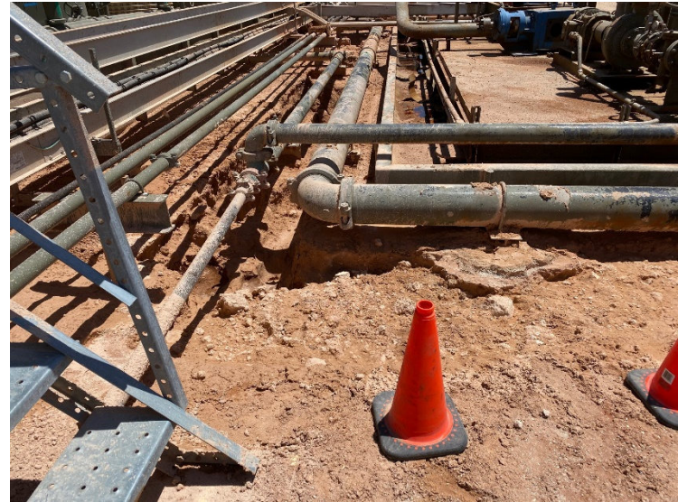
Photograph 6: Hydro-vac work to address staining.
