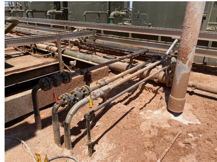
Photograph 4: Hydro-vac work to address staining near BH02.
