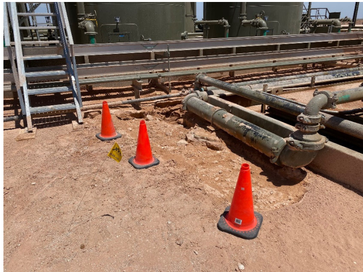
Photograph 7: Western area after hydro-vac work.
