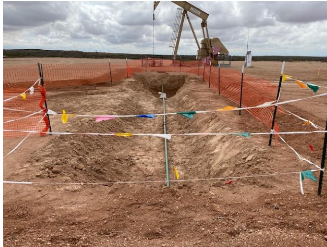
Photograph 11: South view of the final excavation extent.
