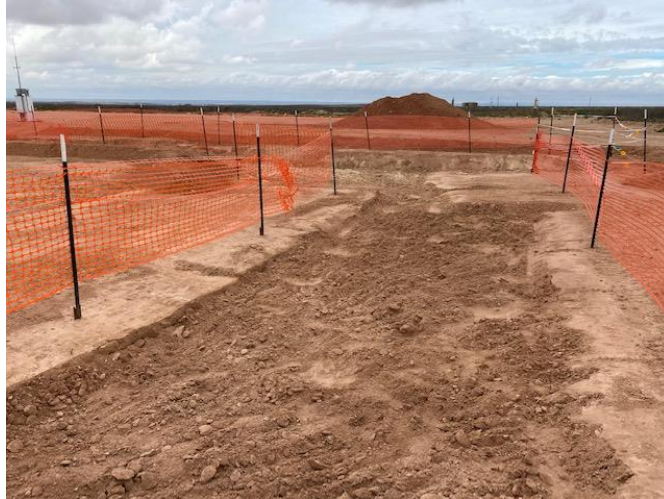
Photograph 10: West view of the final excavation extent.
