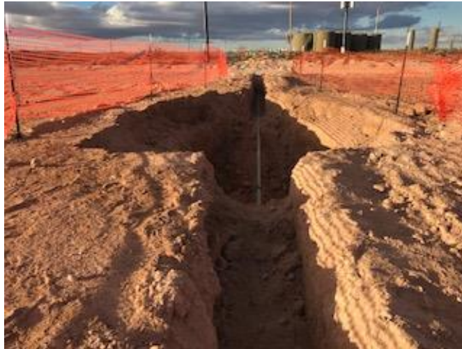
Photograph 4: North view of associated excavation after flowline replacement.
