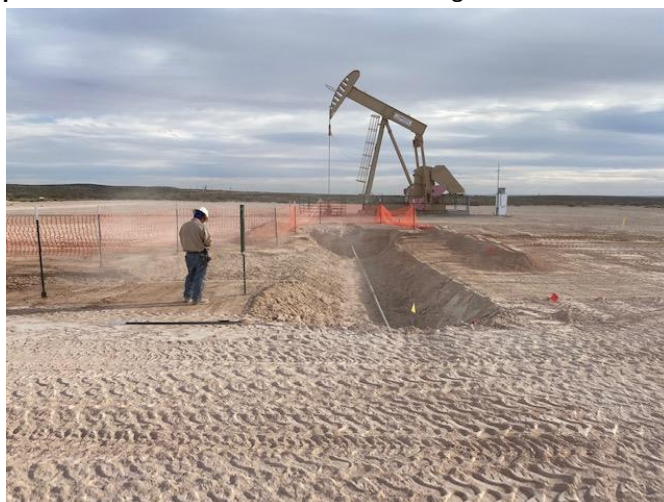
Photograph 8: South view of the Site following additional excavation activities.
