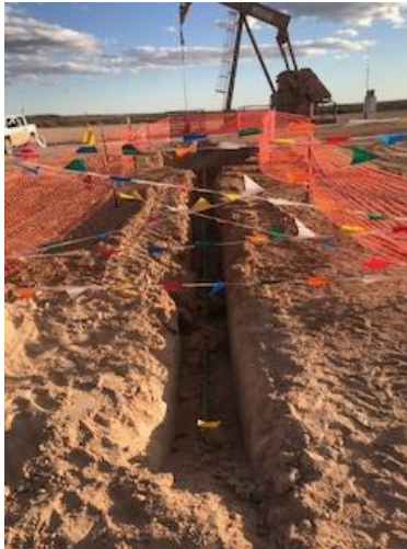
Photograph 5: South view of associated excavation after flowline replacement.
