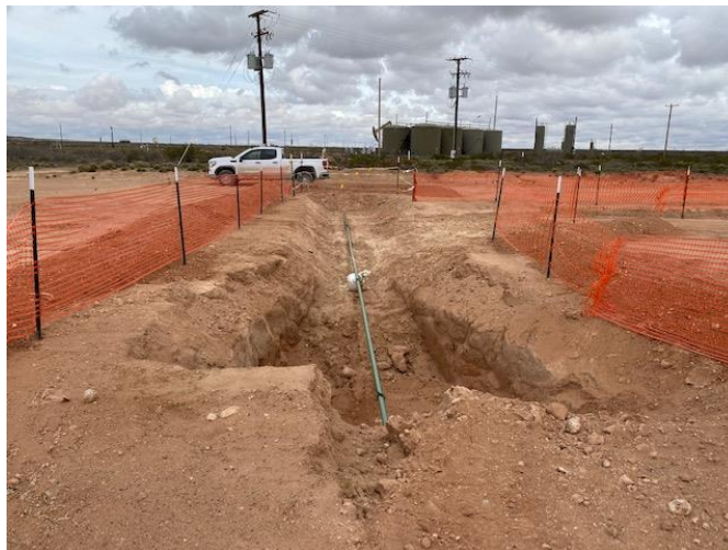
Photograph 12 : North view of the final excavation extent.
