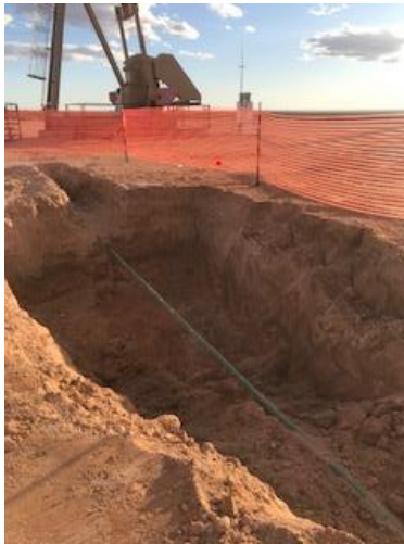
Photograph 6: Southwest view of the associated excavation after flowline replacement.
