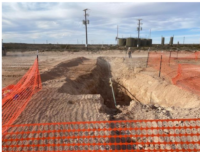
Photograph 9: North view of the Site following additional excavation activities.
