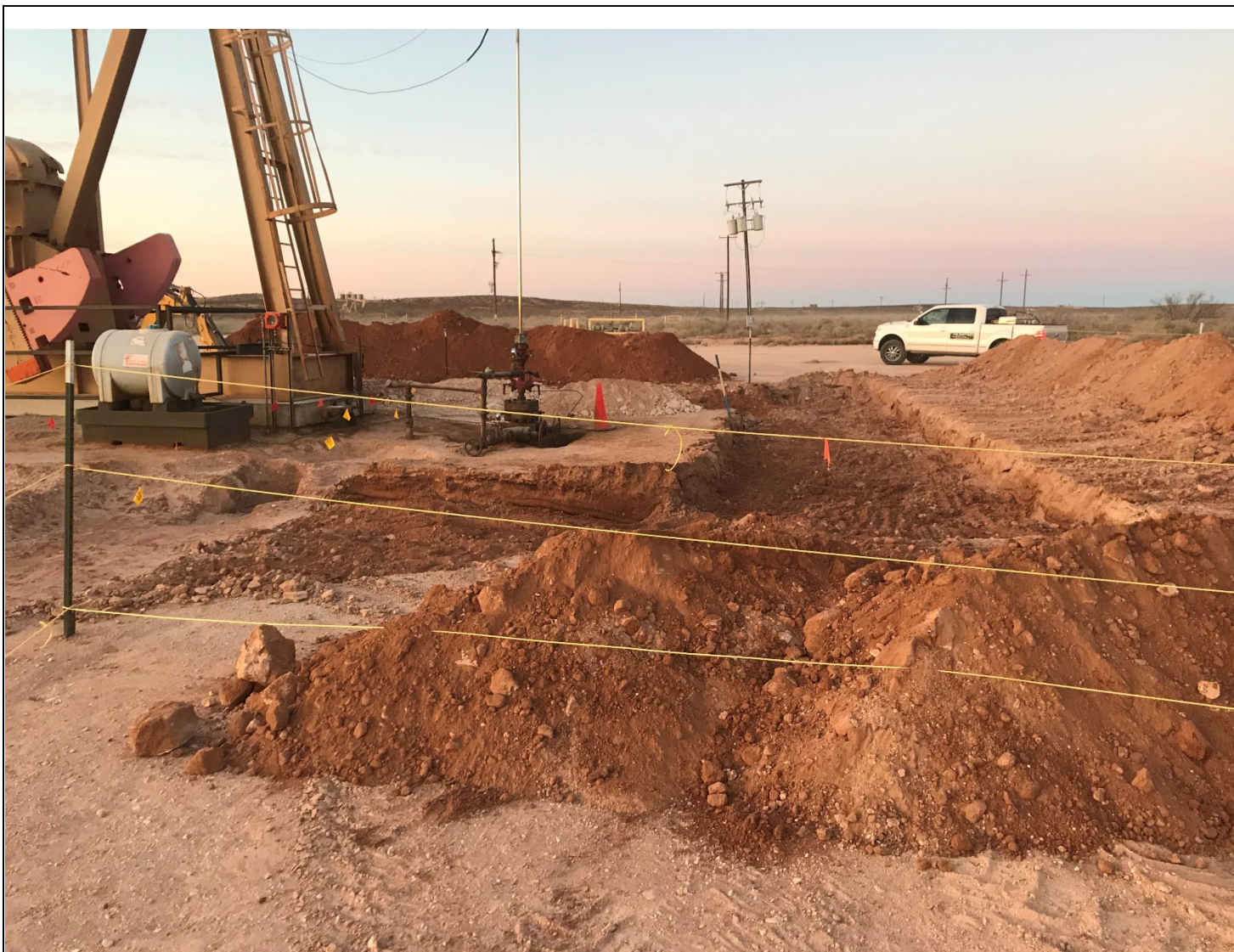
Western north of excavation area.
