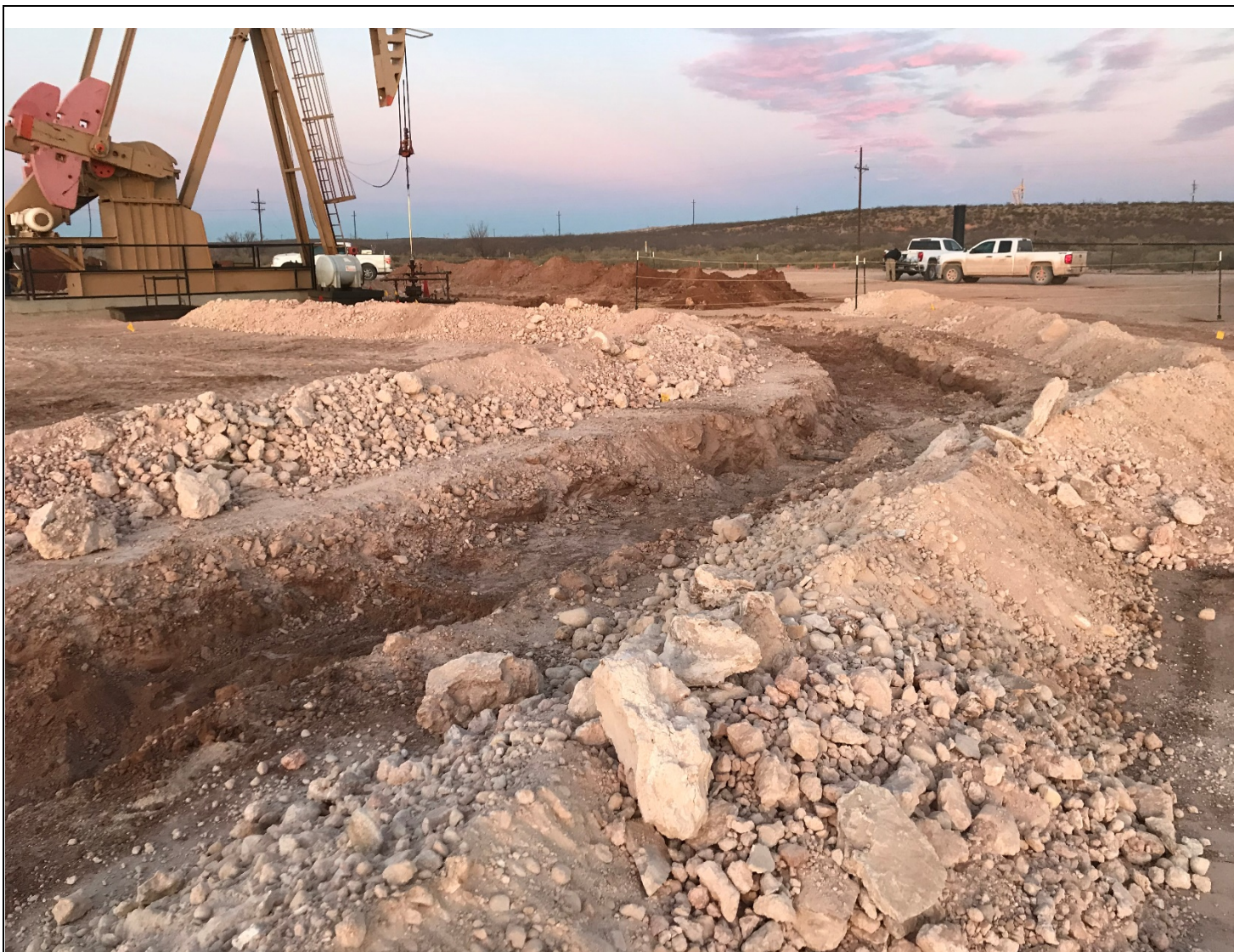
Eastern view of the excavation area.
