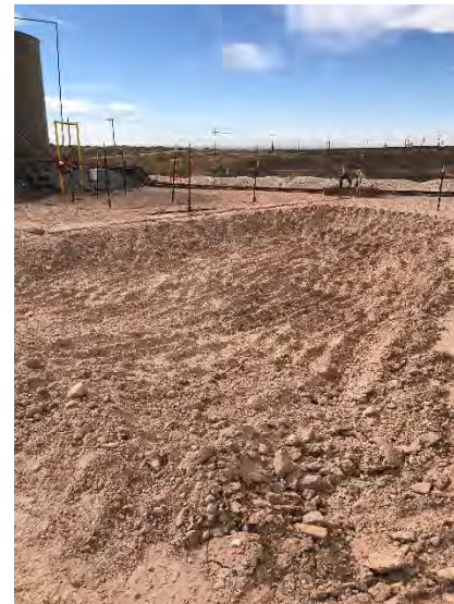
Photograph 4: View of additional on-pad excavation in northwest corner.
