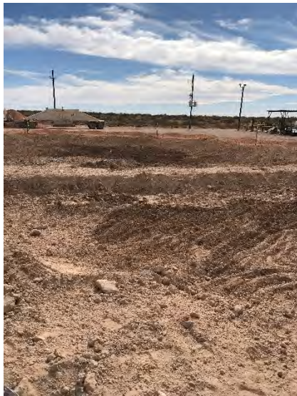
Photograph 3: View of on-pad excavation facing southwest.
