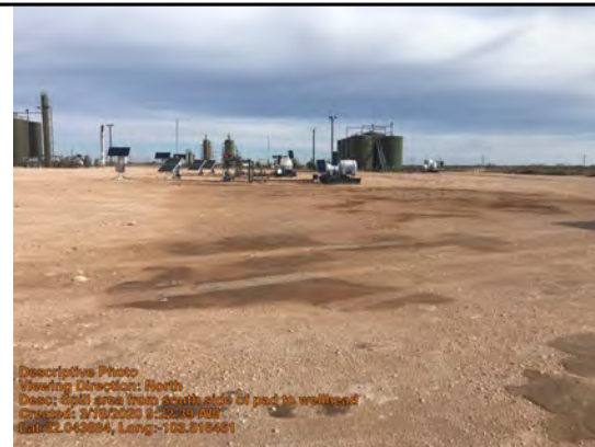
Spill area from south side of pad to wellhead
