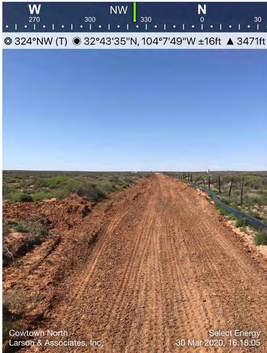
Backfilled and seeded area viewing northwest
