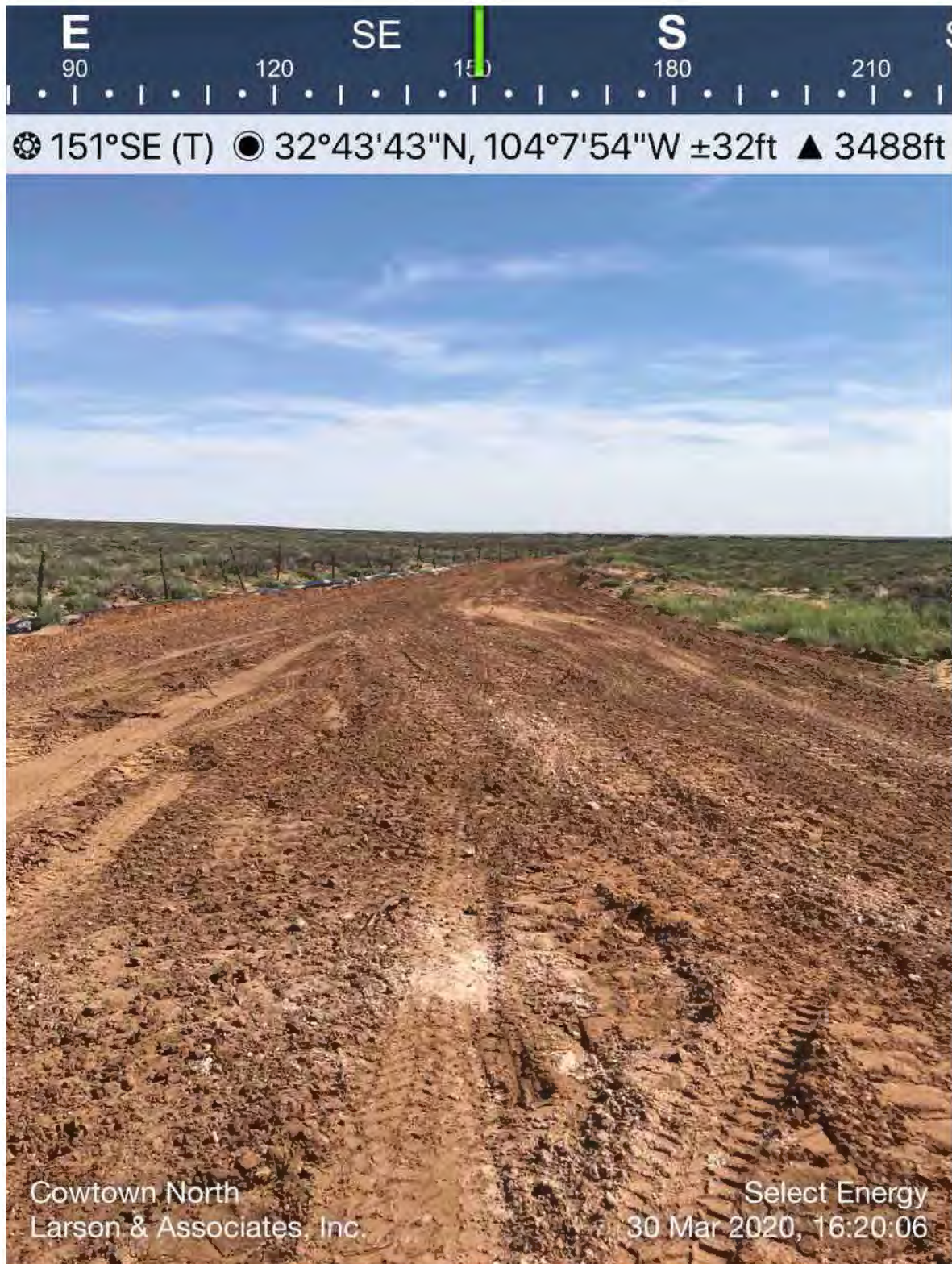
Backfilled and seeded area viewing southeast
