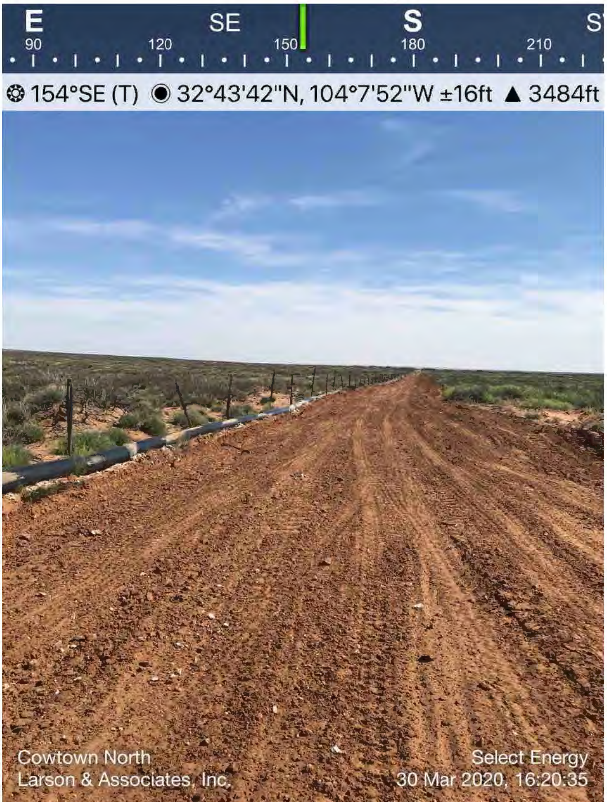
Backfilled and seeded area viewing southeast
