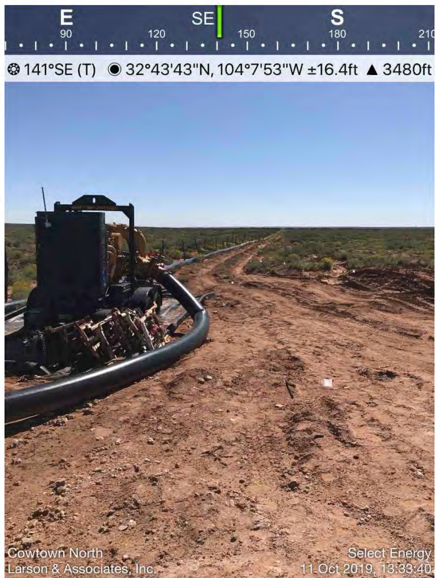
Spill area viewing southeast
