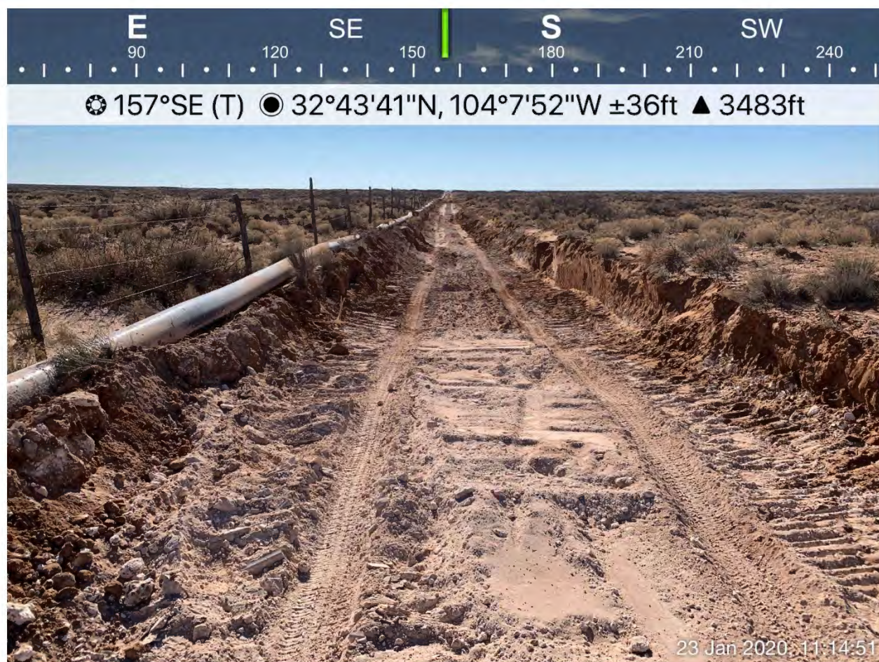
Excavated area viewing south/southeast
