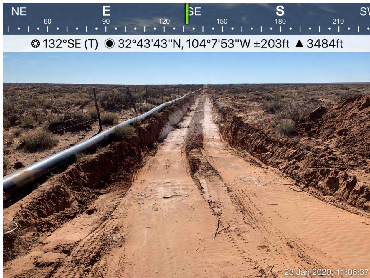
Excavated area viewing southeast
