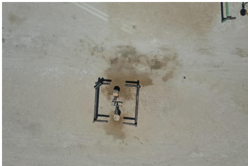
Aerial View of East Impacted Area at Load Out
