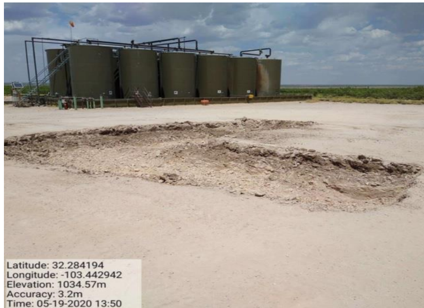
Excavation of West Impacted Area, Facing Northeast
