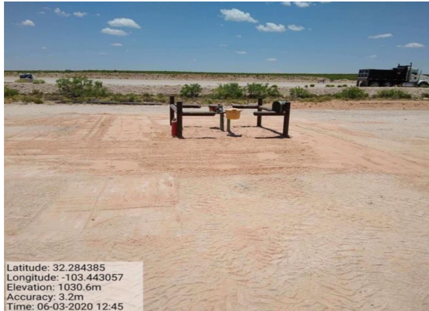
East Excavation Backfilled, Facing North
