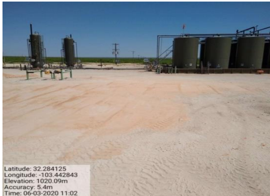
West Excavation Backfilled, Facing North
