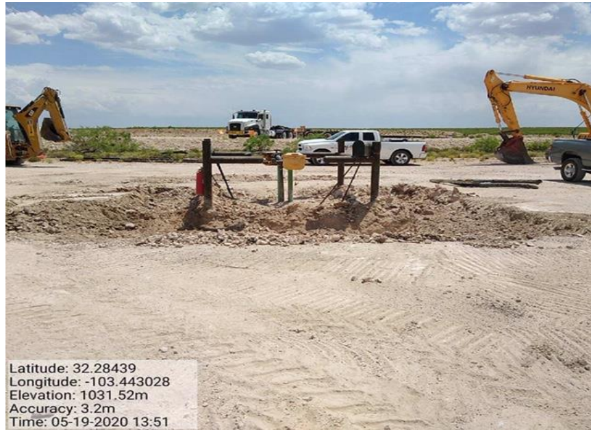
Excavation of East Impacted Area, Facing North
