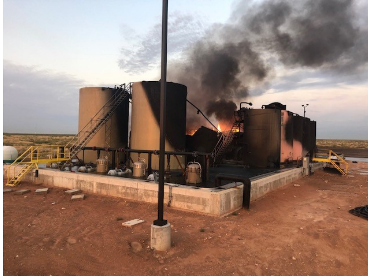
Photograph 1: Damage to tanks and liner due to fire.
