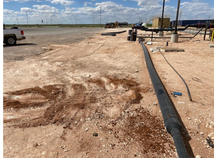
Photograph 6: North facing view release extent.
