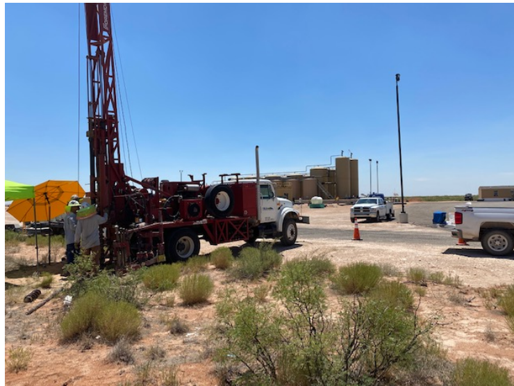
Photograph 7: South facing view of borehole installation.
