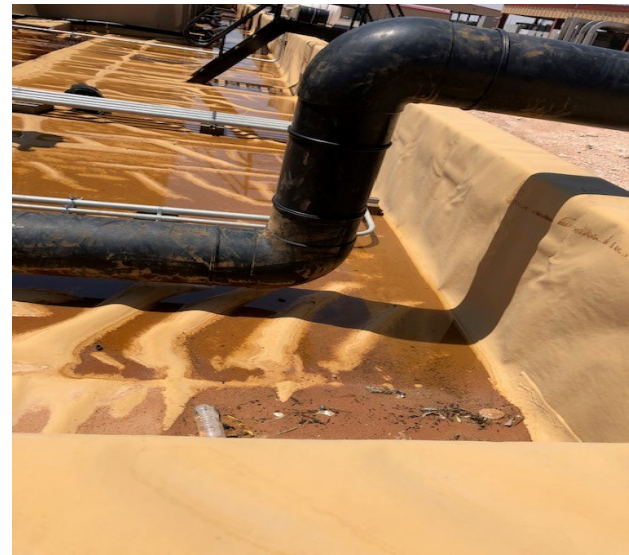
Photograph 4: View of the liner after installation.
