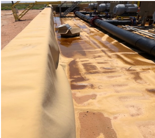
Photograph 3: View of the liner after installation.
