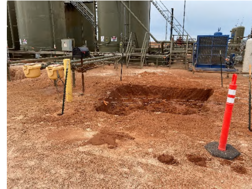
Photograph 6: View of eastern excavation facing north.
