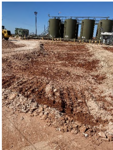
Photograph 3: View of southwestern excavation facing north.
