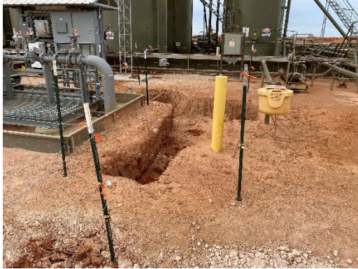
Photograph 5: View of excavation around active production equipment.
