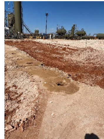
Photograph 4: View of southeastern excavation facing north.
