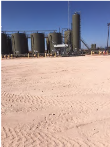
Photograph 7: View of final backfill facing north.
