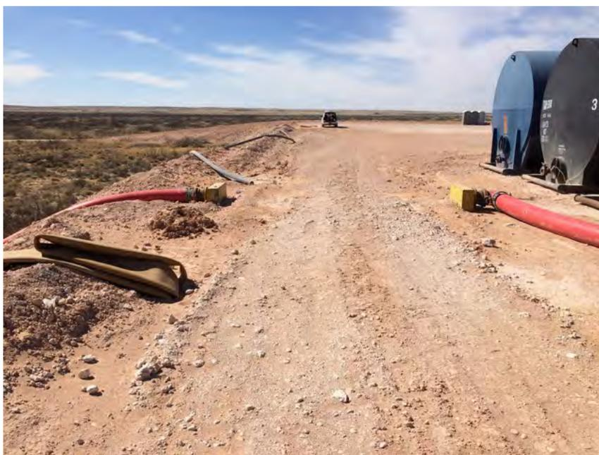
**Figure 2: Photo viewing west near the source (frac tank). Vehicle in photo center background is the western extent of the release. The graded surface is where the removal of impacted surface soils and replacement with clean caliche occurred during initial response. GPS: 32.4151778 N, -103.6033083 W. Date/Time: 2019-02-24 13:19:36**
