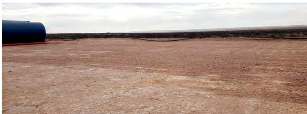
**Figure 1: Graded area shows the eastern half of the release extent that was removed and replaced with clean caliche. Frac tanks are visible photo left. Photo is viewing south-southeast. GPS: 32.4158530 N, -103.6036710 W. Date/Time: 2019-02-08 09:28:16**
