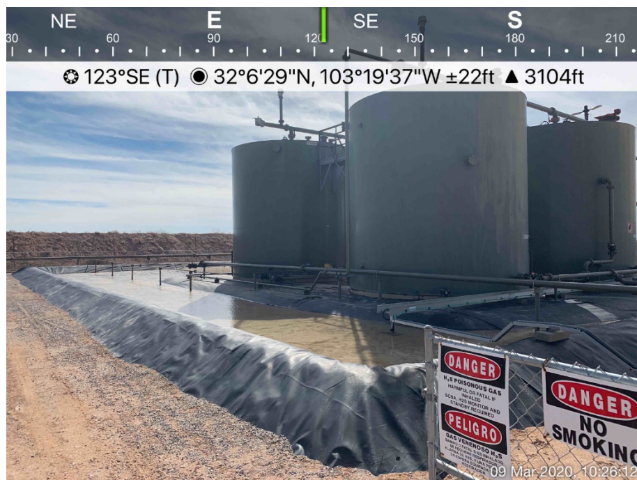
Stormwater contained within lined berm, viewing southeast
