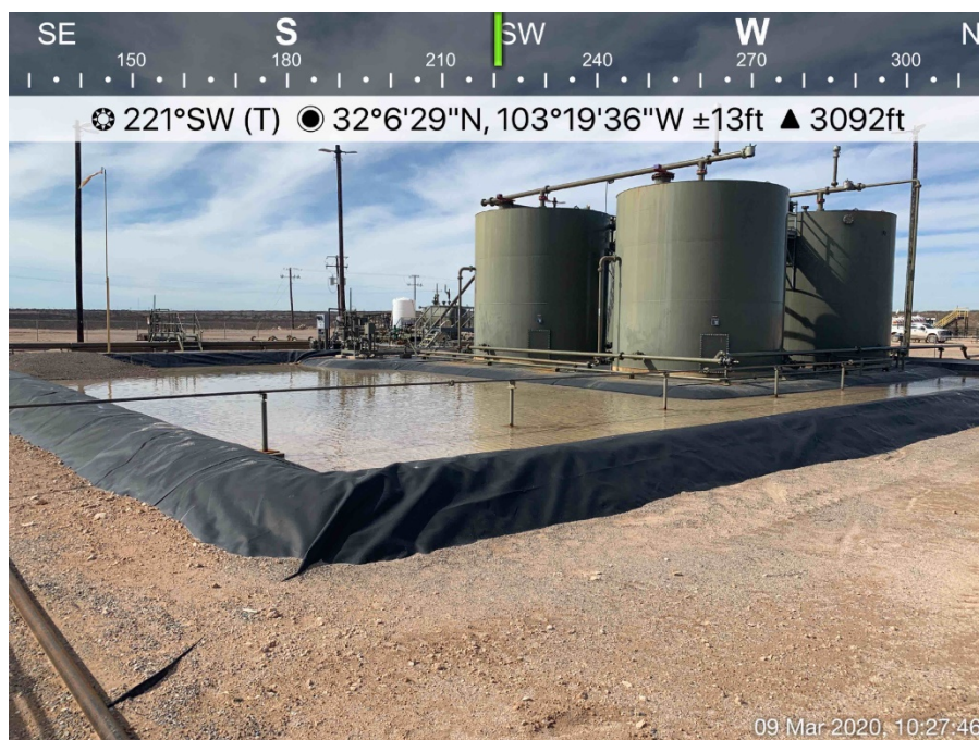
Stormwater contained within lined berm, viewing southwest
