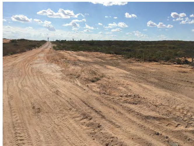
Photograph 3: View of completed backfill along lease road.
