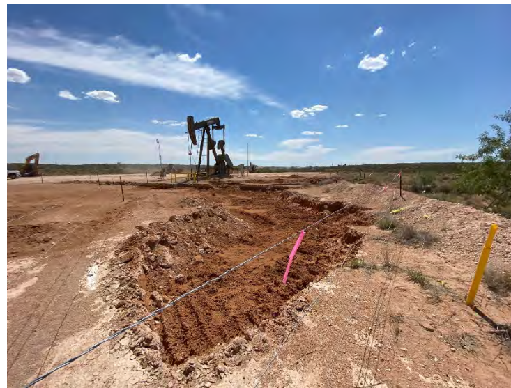
Photograph 10: Western view of excavation on pad.
