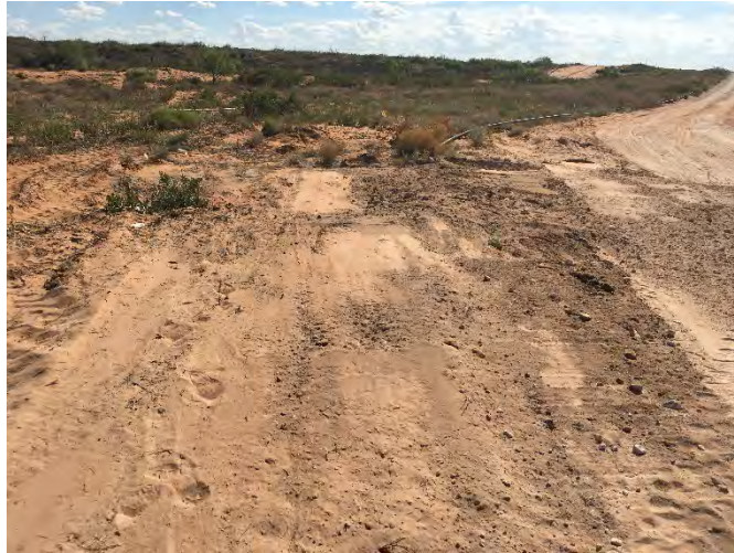
Photograph 2: View of completed backfill along lease road.
