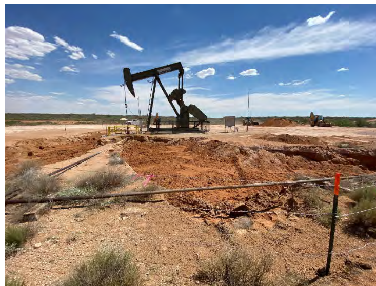
Photograph 12: Southern view of pad excavation.
