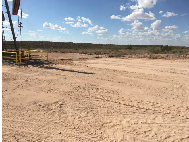
Photograph 1: View of completed backfill on pad.
