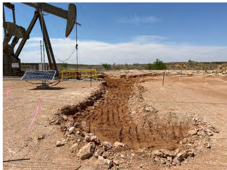
Photograph 11: Northern view of excavation on pad.
