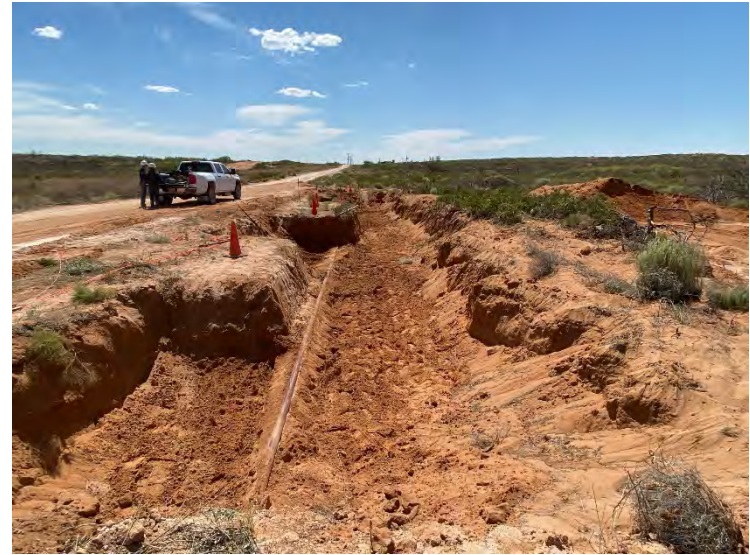
Photograph 6: Western view of excavation in pasture.
