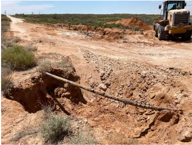
Photograph 5: Northern view of excavation near release point in pasture.
