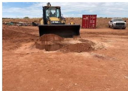
West view of the Site during delineation activities.
