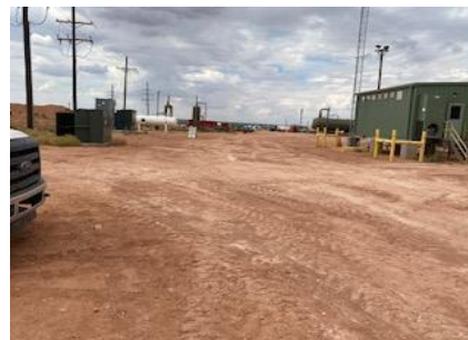
North view of the Site following delineation activities.
