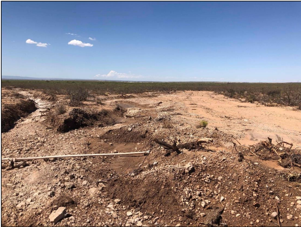
PHOTO 25: View of excavation toward HA-3, facing northwest. 9/26/2019
