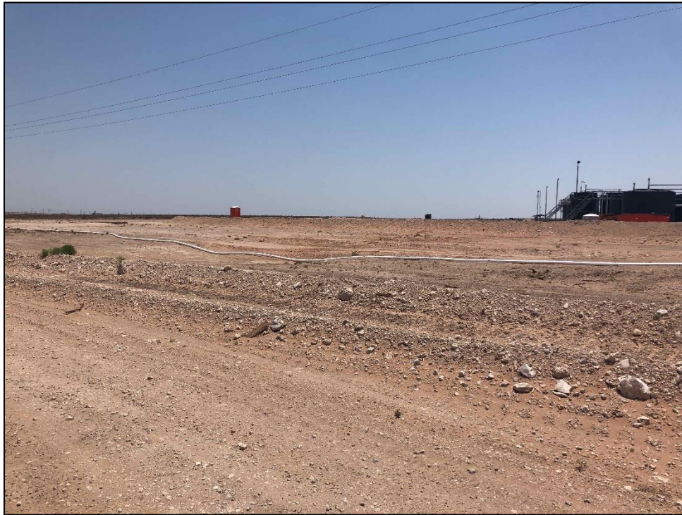
PHOTO 33: View of completed remediation, facing east. 6/22/2020
