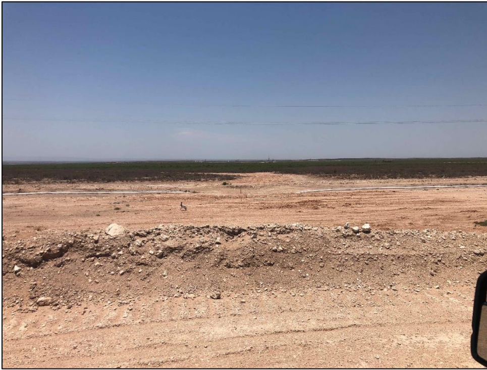
PHOTO 30: View of completed remediation, facing west. 6/22/2020
