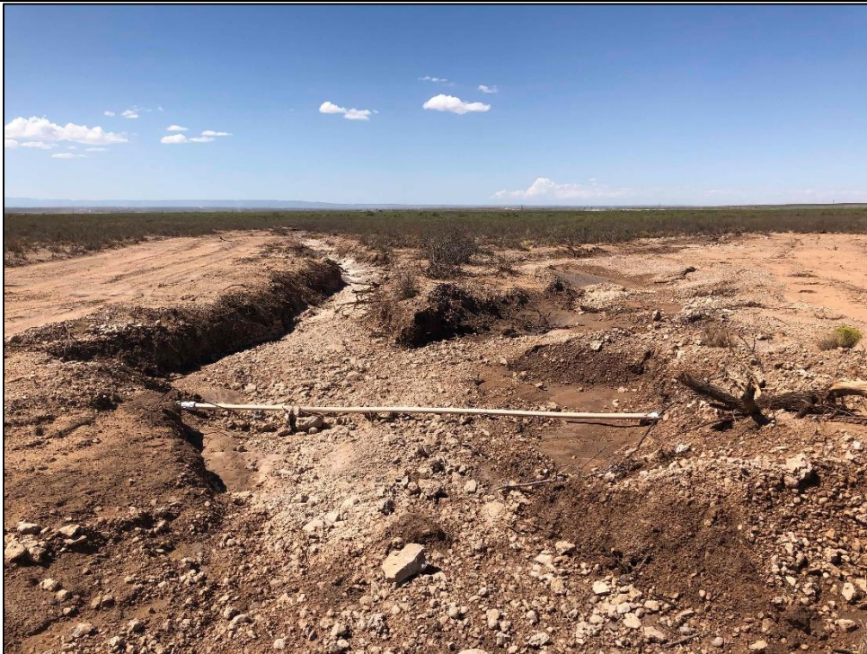
PHOTO 24: View of excavation, facing west. 9/26/2019
