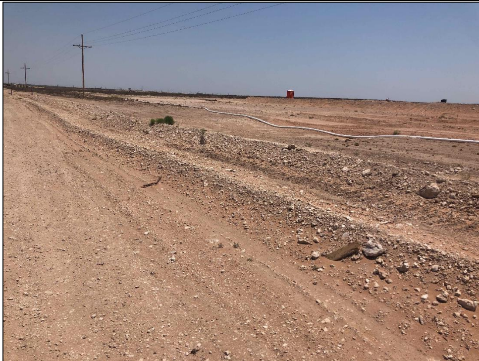
PHOTO 21: View of completed remediation, facing northeast. 6/22/2020
