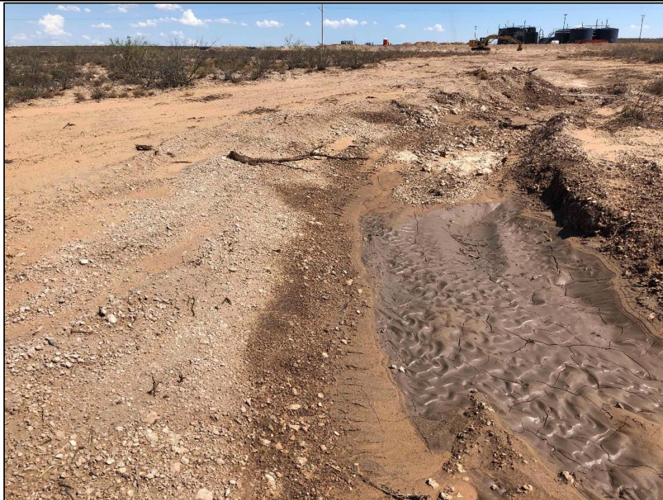
PHOTO 32: View of excavation facing HA-4, facing east. 9/26/2019
