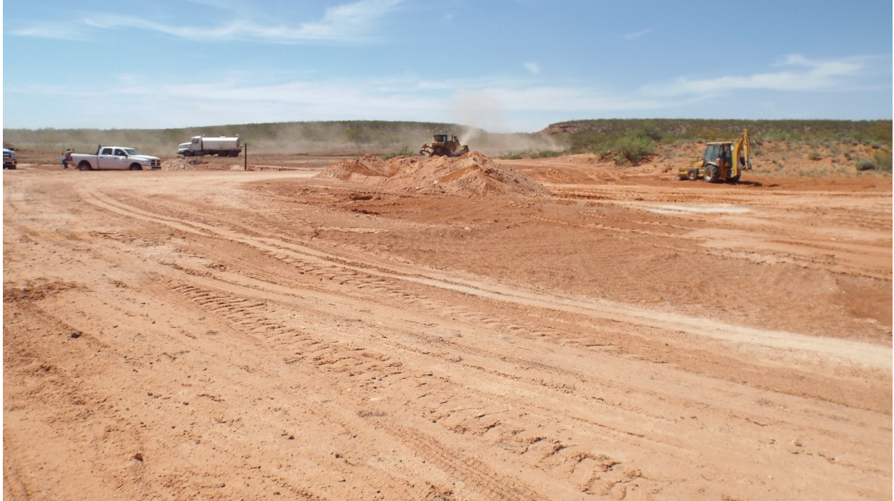
Capping former reserve pit with topsoil, compacting, top photo, facing NW 6/2/2014
