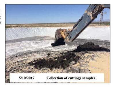
As shown in the table below, laboratory analysis of the cuttings sample meets in-place closure target concentrations found in Table II of 19.15.17.13 NMAC without mixing with 3 parts soil/earth. A robust centrifuge and closed loop system were used at each of these wells to
