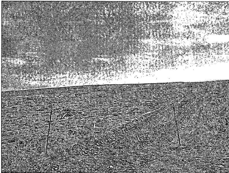
Photo 2. Access road ripped, re-seeded and fenced.
