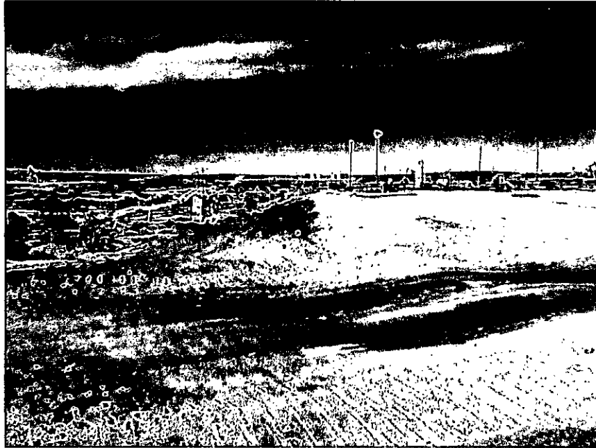
West side of IR. Some material was placed on south where cut is located. A 3:1 slope with berm to prevent run off was constructed.
