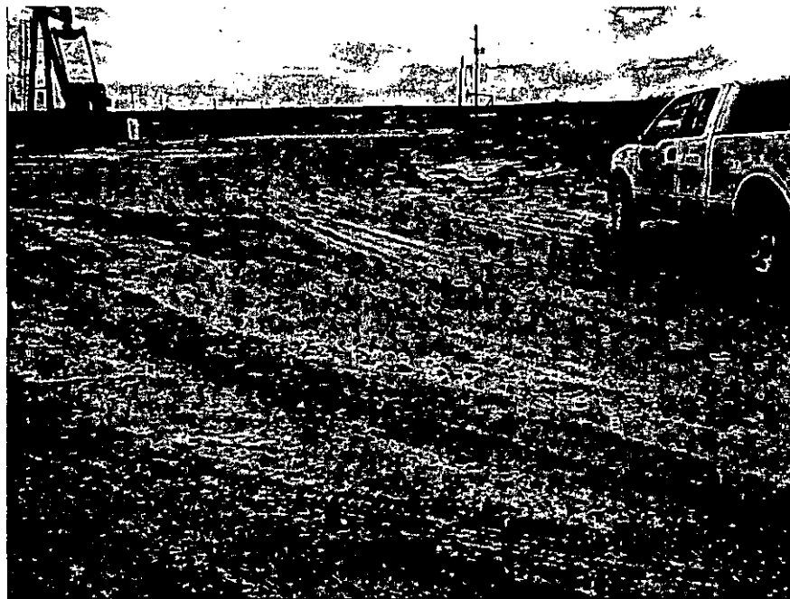
NORTH EDGE OF WELL PAD RIPPED ACROSS SLOPE AND BERMED
