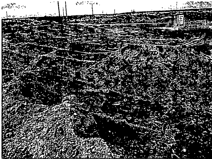
EAST EDGE OF WELL PAD WITH LARGE RIPS TO PREVENT EROSION.
