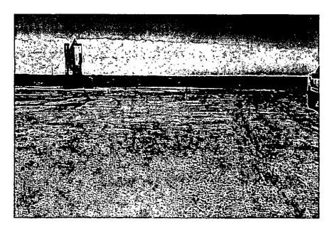
IR as per planned in AAPD plus reclamation south of lease road running through well pad. Location bermed, slopes greater than 3:1, rips across the slope, corners rounded off to reclaim areas not needed for daily operations.
