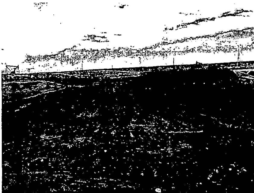
RECLAMATION ON NORTH WITH GREATER THAN 3:1. RIPS ACROSS THE SLOPE. WELL PAD TAPERS BACK INTO THE CUT TO PREVENT EROSION ON DOWNSLOPE.
