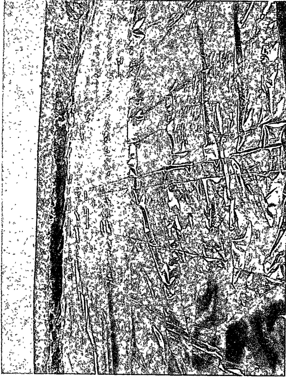
20 mil impervious cap over drilling pit.
