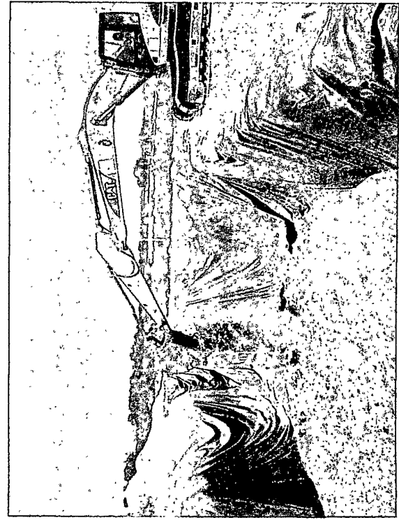
Placing mud in burial pit after stiffened with dry soil.
