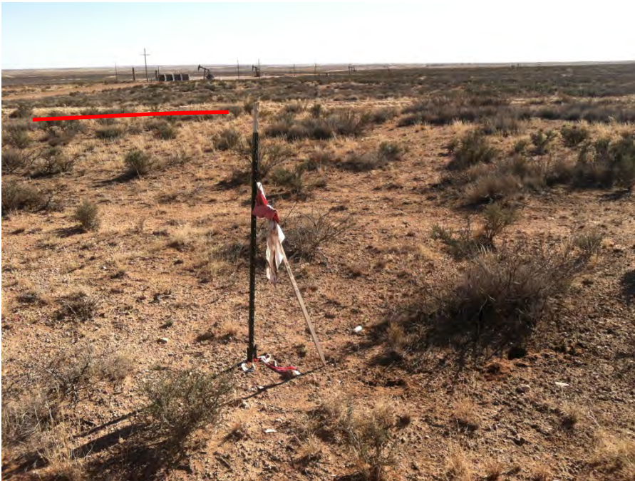
View south from staked location showing re-vegetation along pipeline trace (above red line) and small swale south of pipeline.
