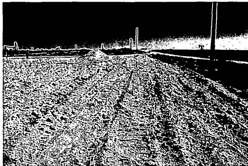
IR as per planned in AAPD plus reclamation north and east sides. Location bermed, slopes greater than 3:1, rips across the slope, corners rounded off to reclaim areas not needed for daily operations.
