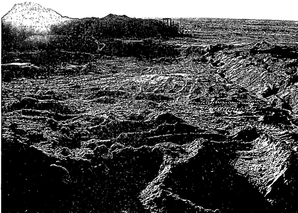
Photograph No. 12 – Backfilling with excavated stockpiled material over top soil cushion layer
