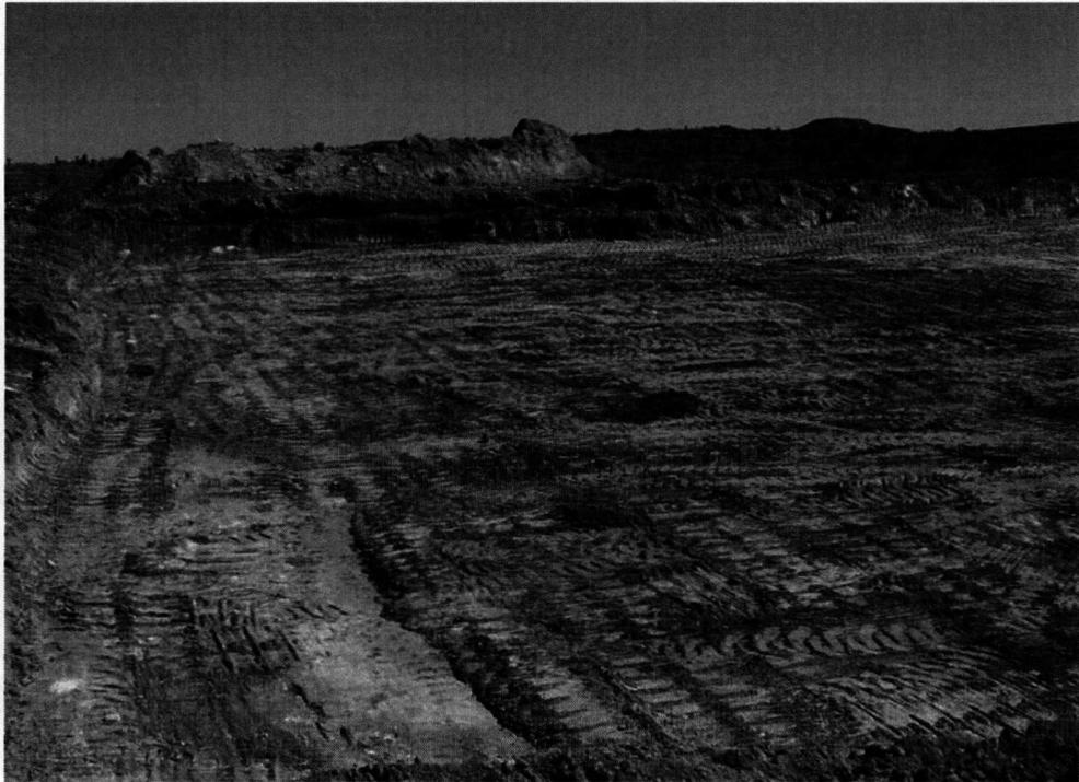
Photograph No. 9 – Finished layer of top soil cushion material for polyethylene layer
