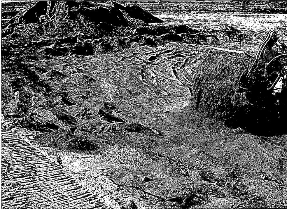
Photograph No. 11 – Placing top soil cushion over polyethylene liner
