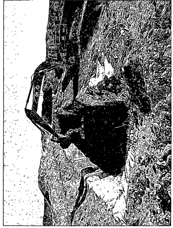
Drilling mud being placed into burial pit.
