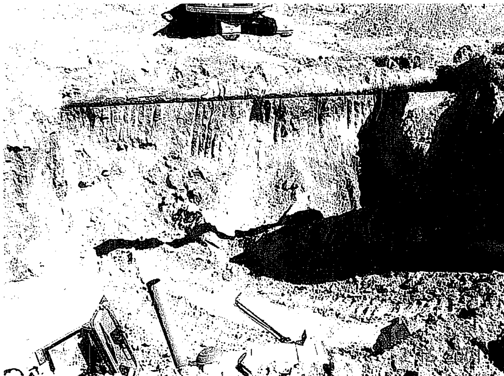
View facing east showing widespread hydrocarbon staining on walls and floor of excavation
