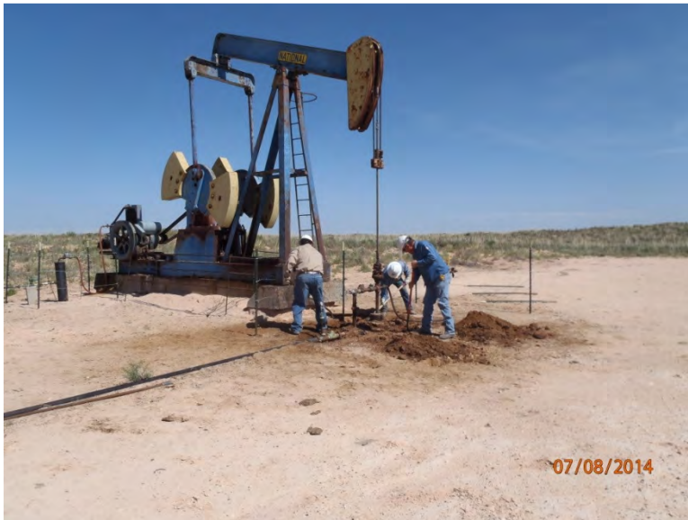
Shoveling release around well head, facing north-west 7/8/14
