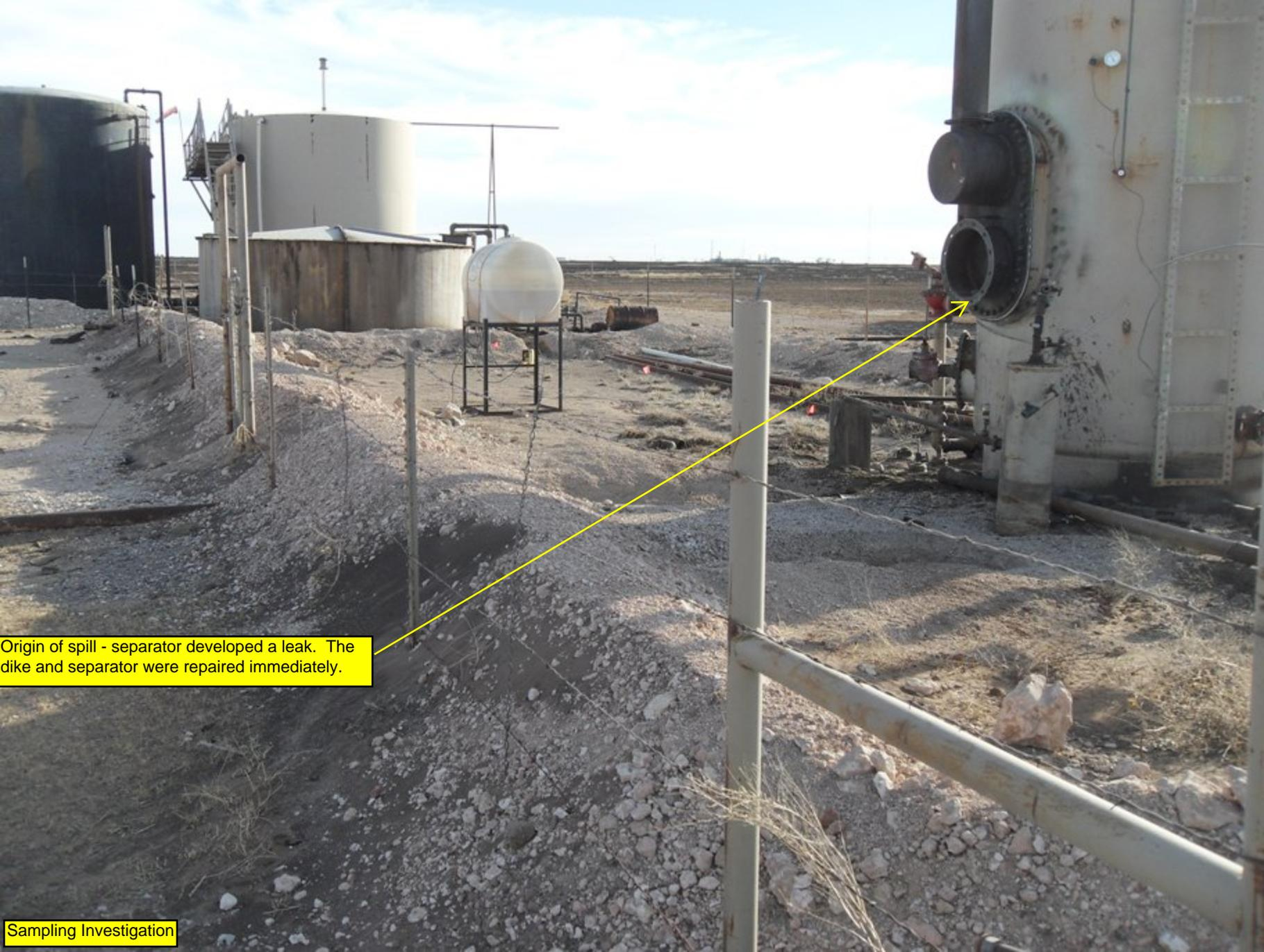
Origin of spill - separator developed a leak. The dike and separator were repaired immediately.
