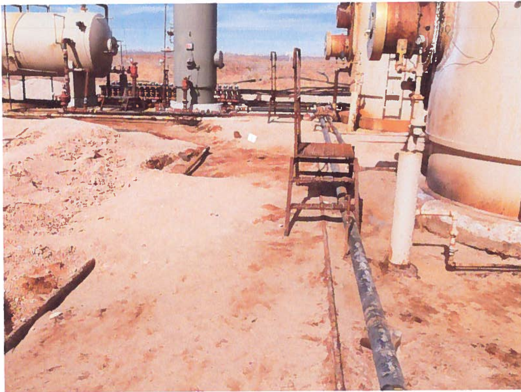
View North – Area of AH-3
