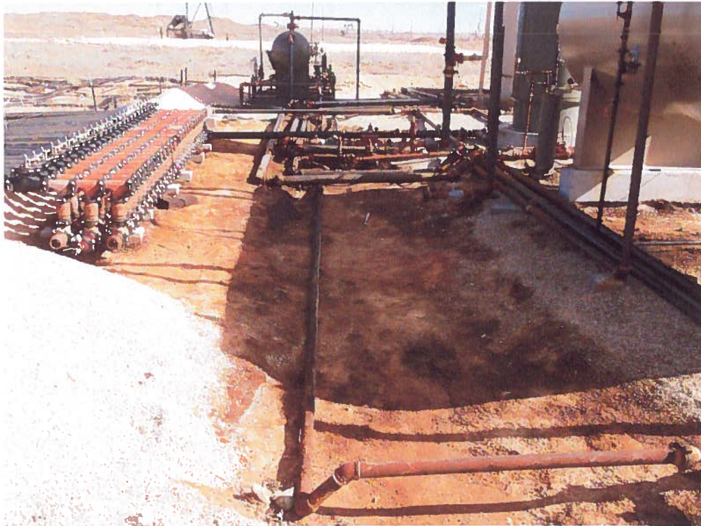
View East – Area of AH-1
