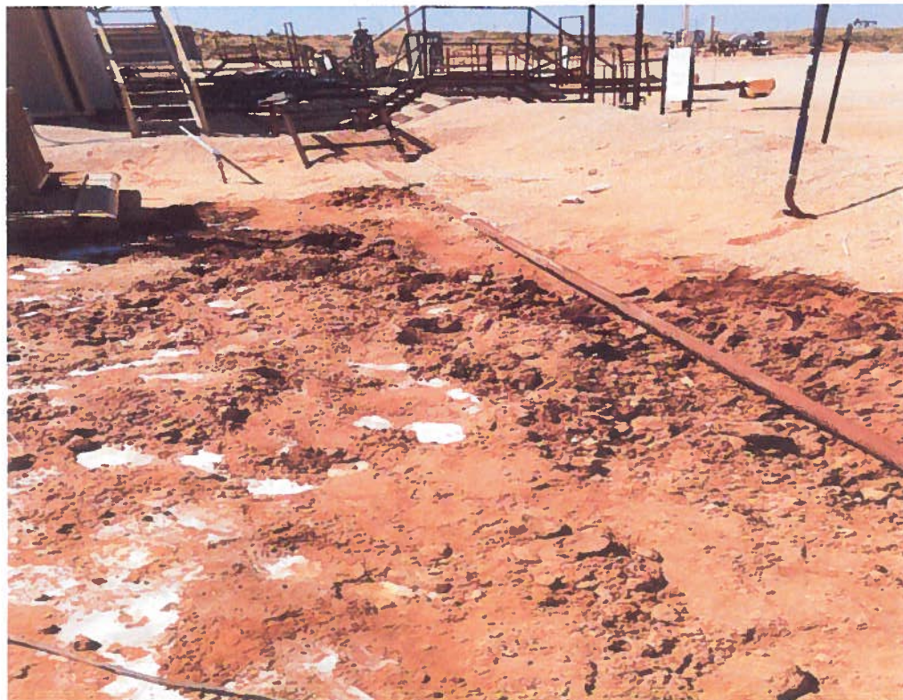
View of Soil Remediation and Micro-Blaze Treatment
