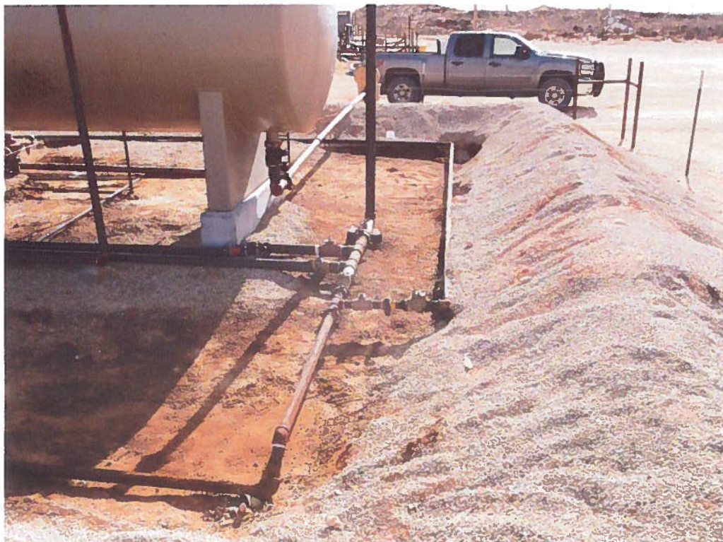
View South – Area of AH-2
