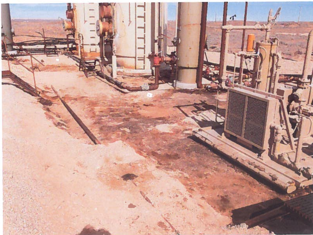
View North – Area of AH-4
