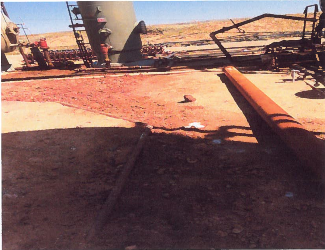
View of Soil Remediation and Micro-Blaze Treatment
