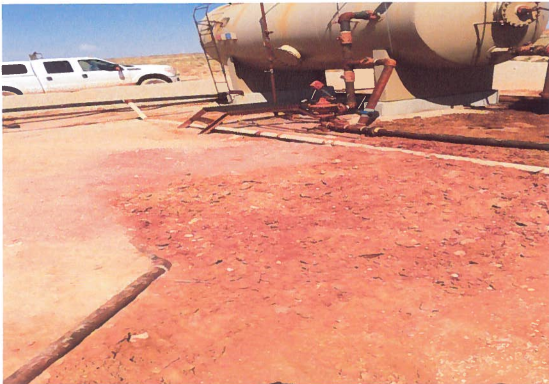
View of Soil Remediation and Micro-Blaze Treatment
