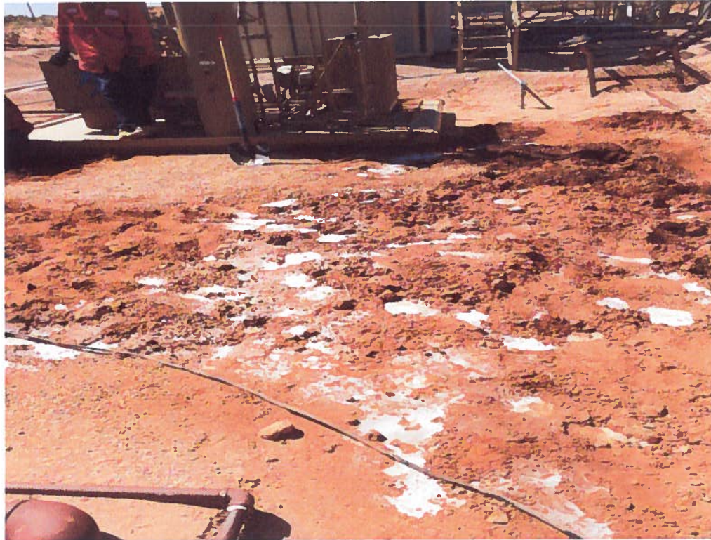
View of Soil Remediation and Micro-Blaze Treatment
