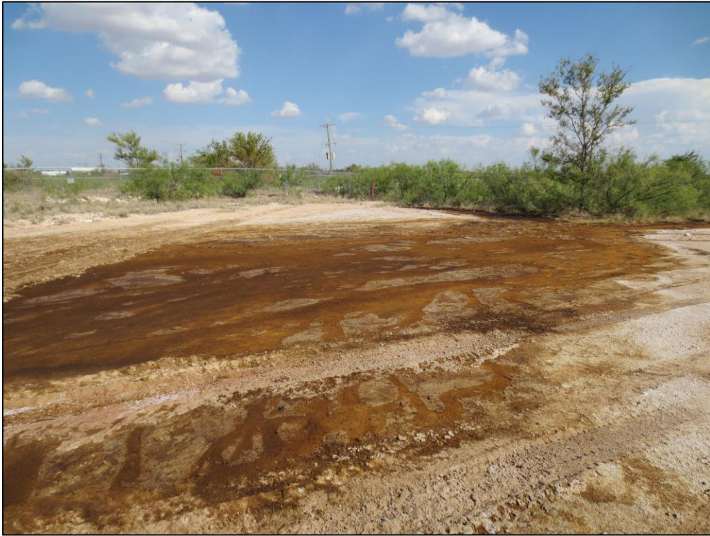
Release area on pad looking Southeast
