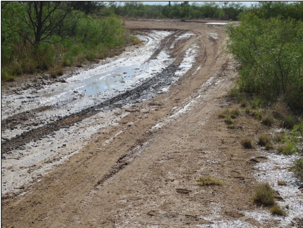
Lease road looking West
