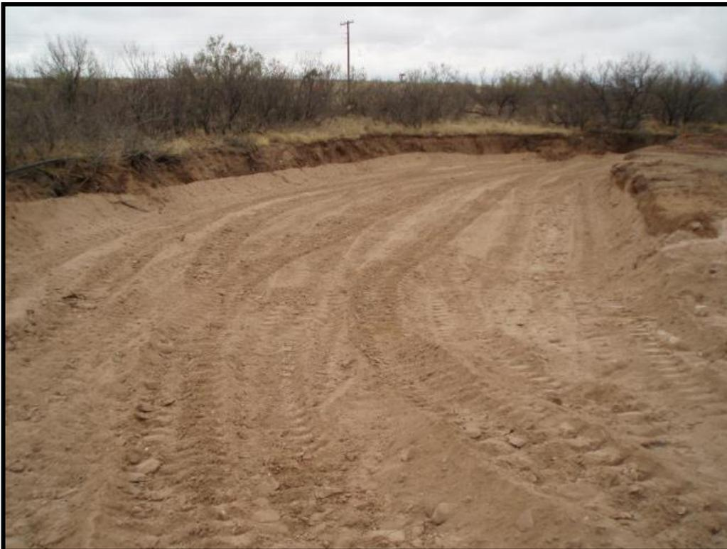
Excavation Backfilled to 4' bgl Facing SE
