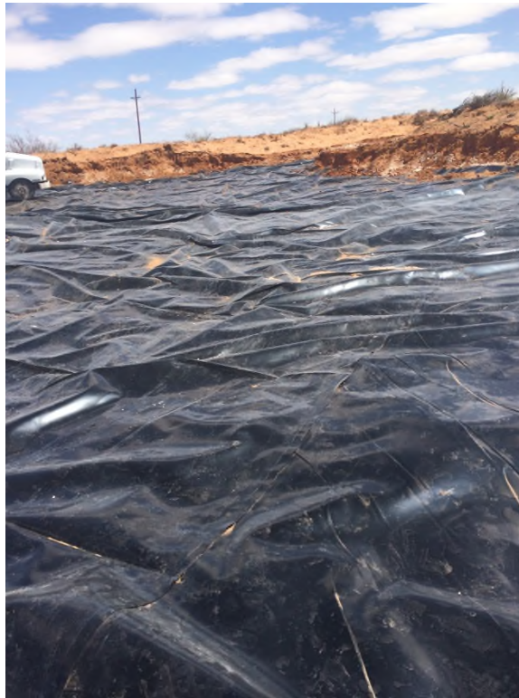
View North – Lined area of the South Spill
