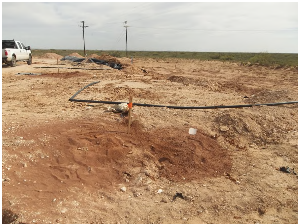
View South – Area of BH-1 and BH-2
