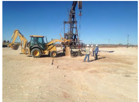
Backfilling area surrounding wellhead, facing northwest
