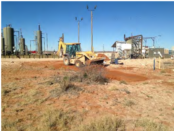
Backfilling 3' excavation, facing northwest 2/12/2016
