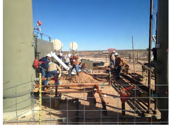
Removing soil around compressor area by hand, facing north 2/8/2016
