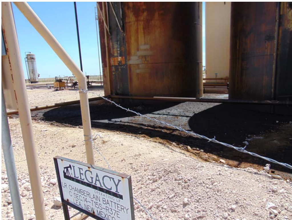
Photograph #1- Release with in containment berm.
