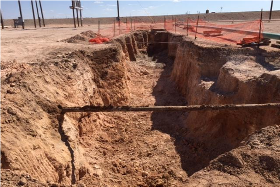
View of the excavated release point.
