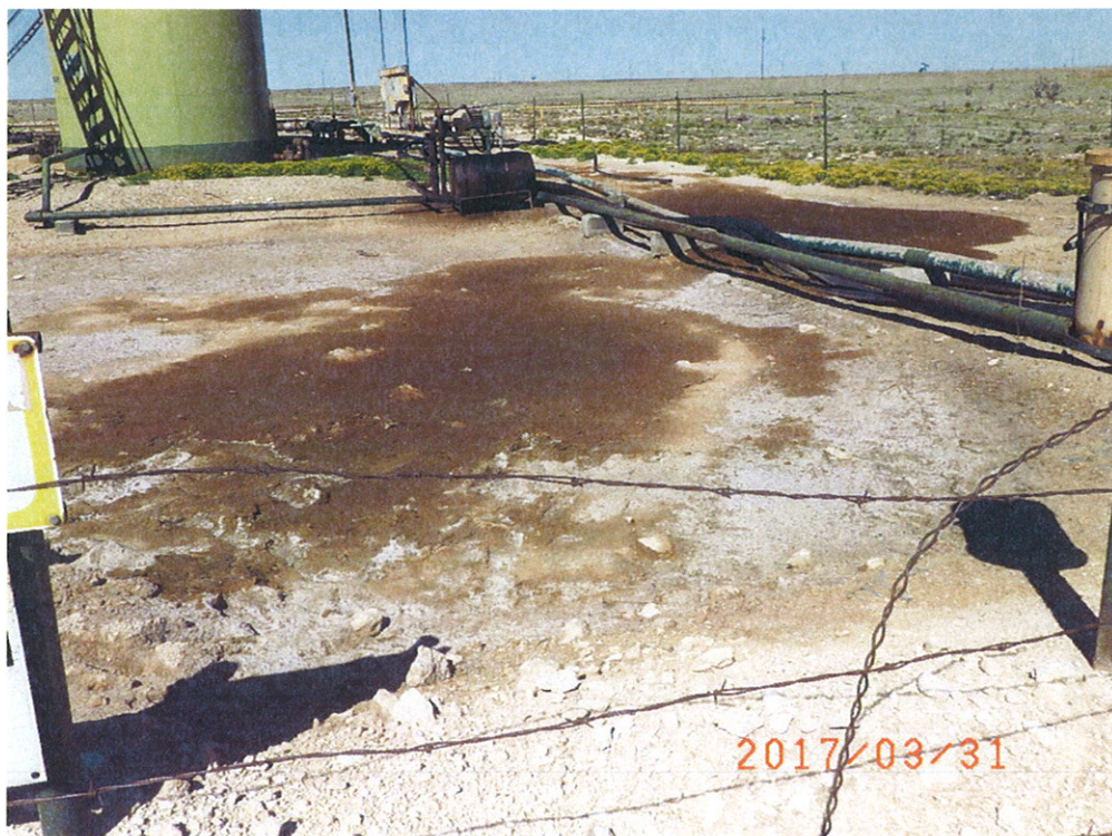
Spill Area North and East of Battery Viewing Northwest
