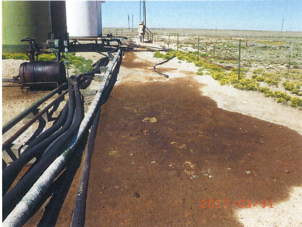
Spill Area North of Battery Viewing West
