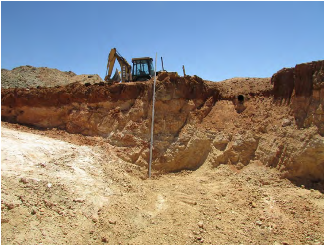
Sample Collection from Southeast Side, April 28, 2016 Note: Approximate depth 11 feet
