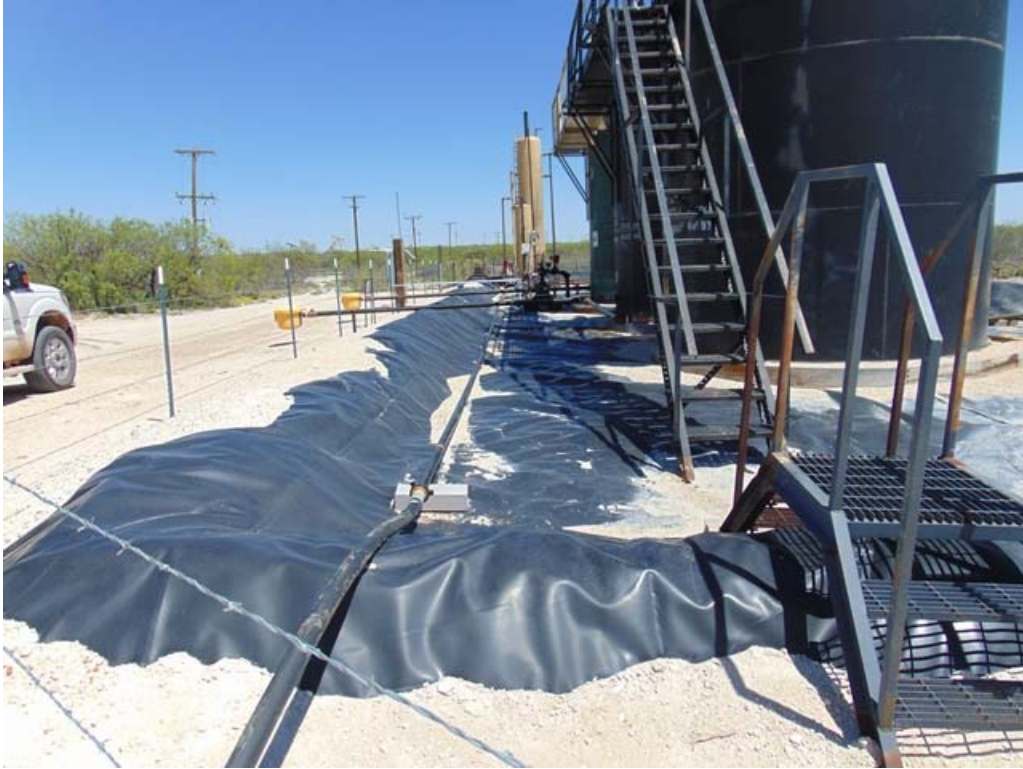
Photograph #5 – Rebuilt tank battery with new liner
