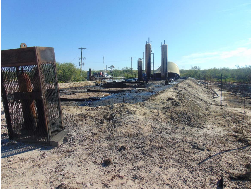
Photograph #1 – Tank battery struck by lightning
