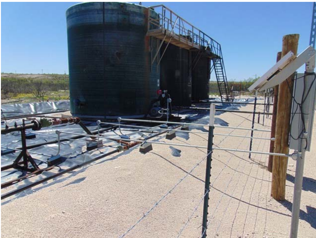
Photograph #6 – Rebuilt tank battery with new liner
