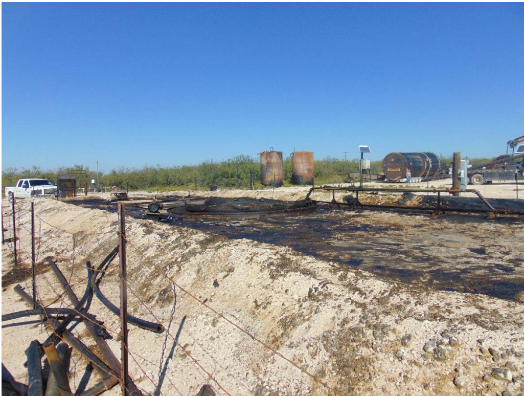
Photograph #2 – Tank battery struck by lightning
