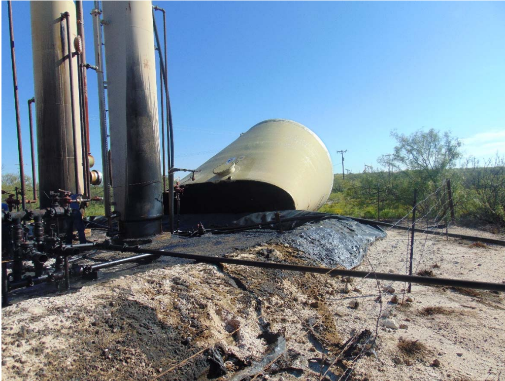
Photograph #3 – Tank battery struck by lightning
