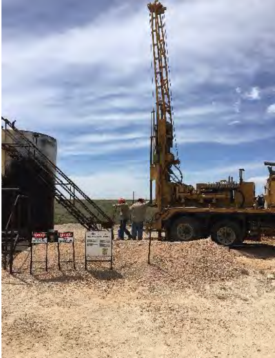
Photo 1: Hollow Stem Auger Rig set up on V1 (vertical delineation location) inside Tank Battery
