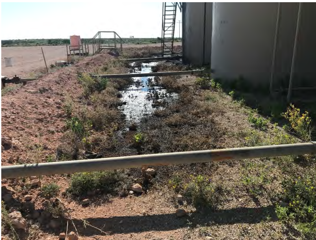
Red Tank 24 Fed 1 & 2 CTB - Release (Looking East)
