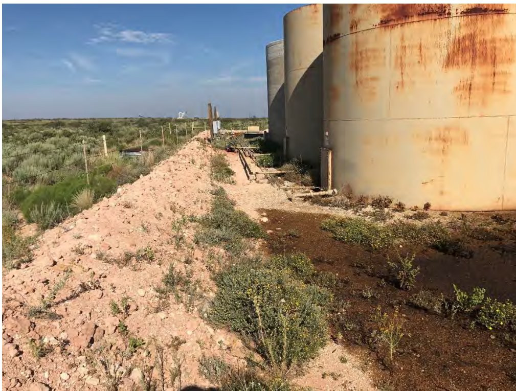
Red Tank 24 Fed 1 & 2 CTB – Release (Looking West)
