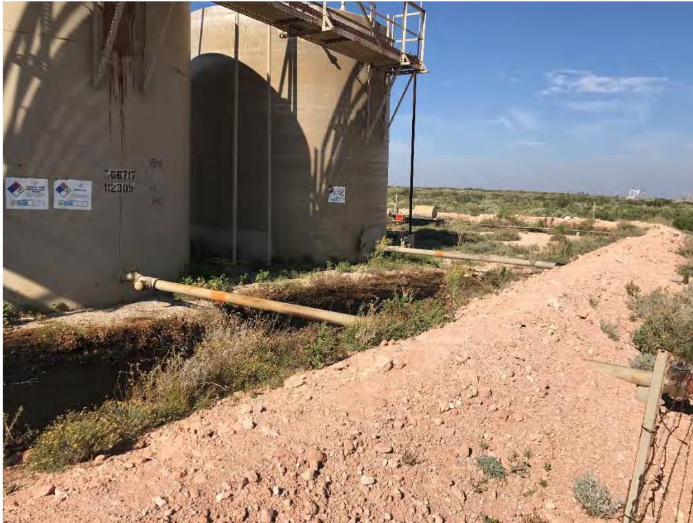
Red Tank 24 Fed 1 & 2 CTB - Release (Looking Southwest)
