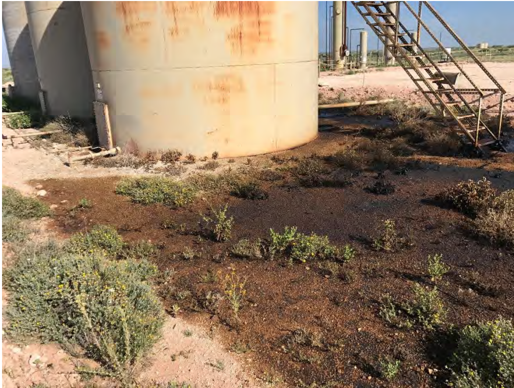
Red Tank 24 Fed 1 & 2 CTB – Release (Looking Northwest)
