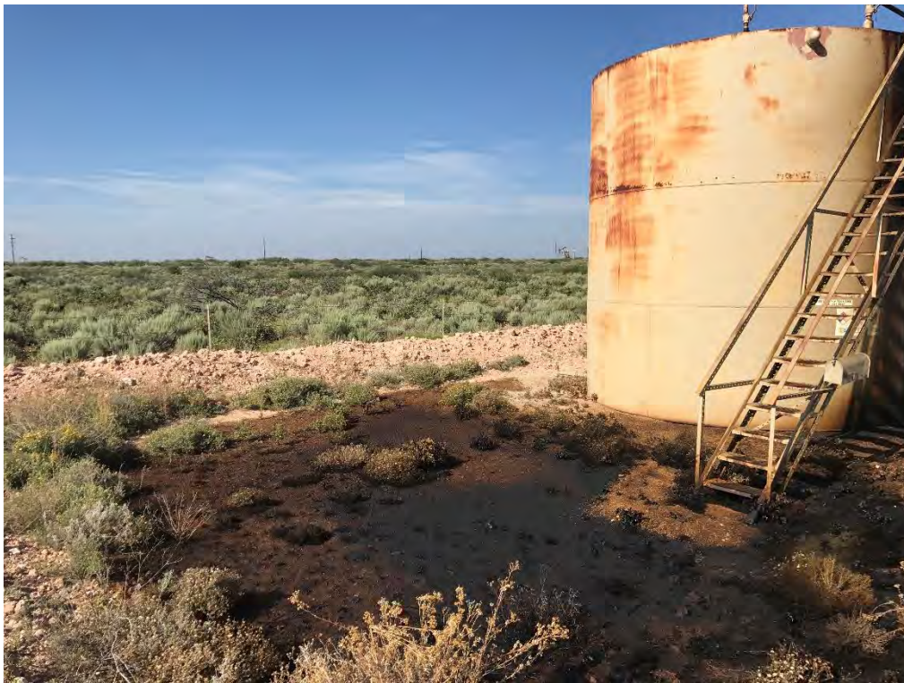
Red Tank 24 Fed 1 & 2 CTB – Release (Looking Southwest)
