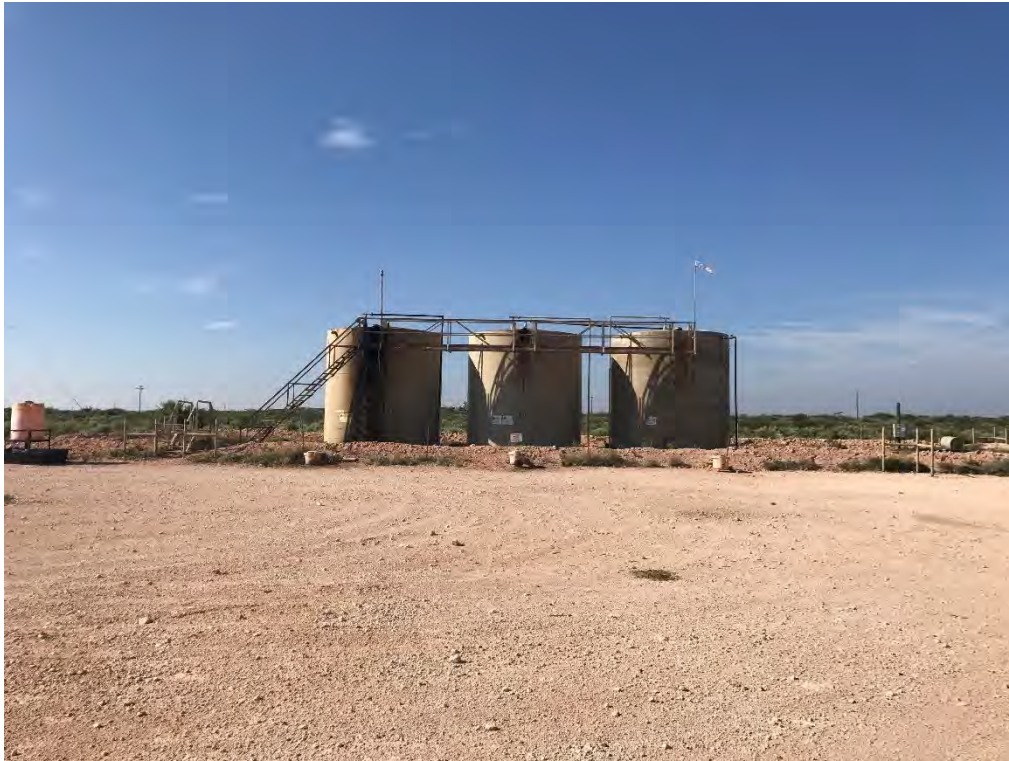
Red Tank 24 Fed 1 & 2 CTB - Release Site (Looking South)
