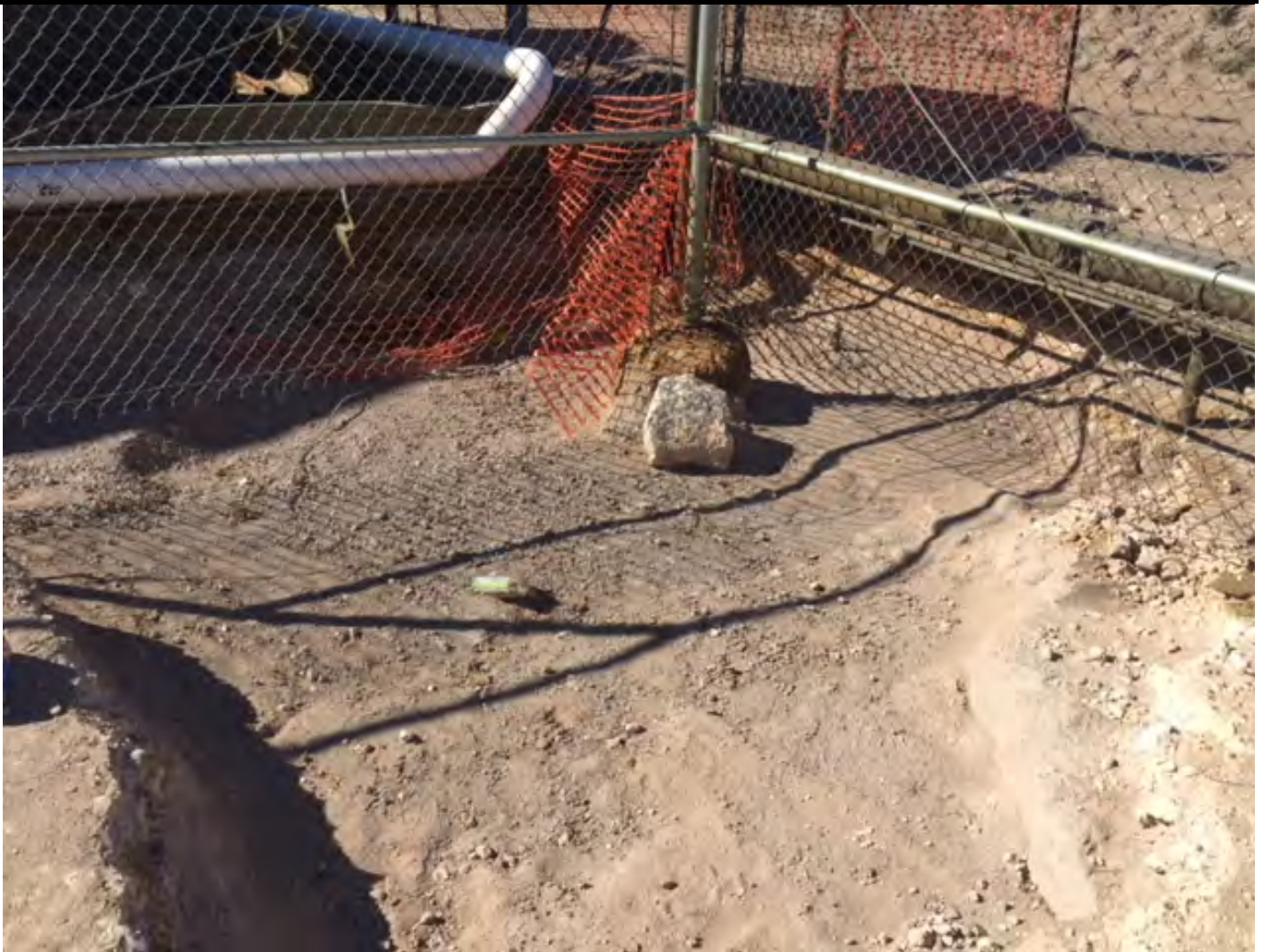
Photo 6: View of portion of the excavated area, facing northwest.
