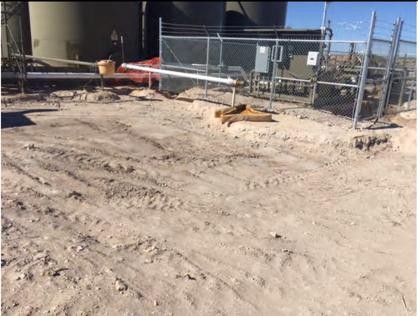
Photo 4: View of portion of the excavated area, facing northwest.
