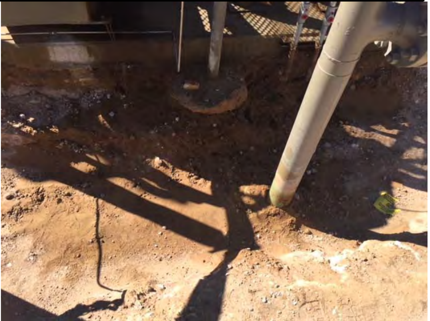
Photo 8: Representative view of impacted soil remaining in-situ adjacent to the LACT unit and high-pressure pipelines.
