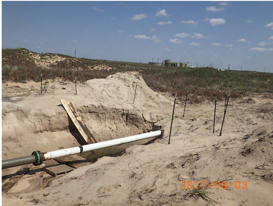
Site Viewing Southeast
