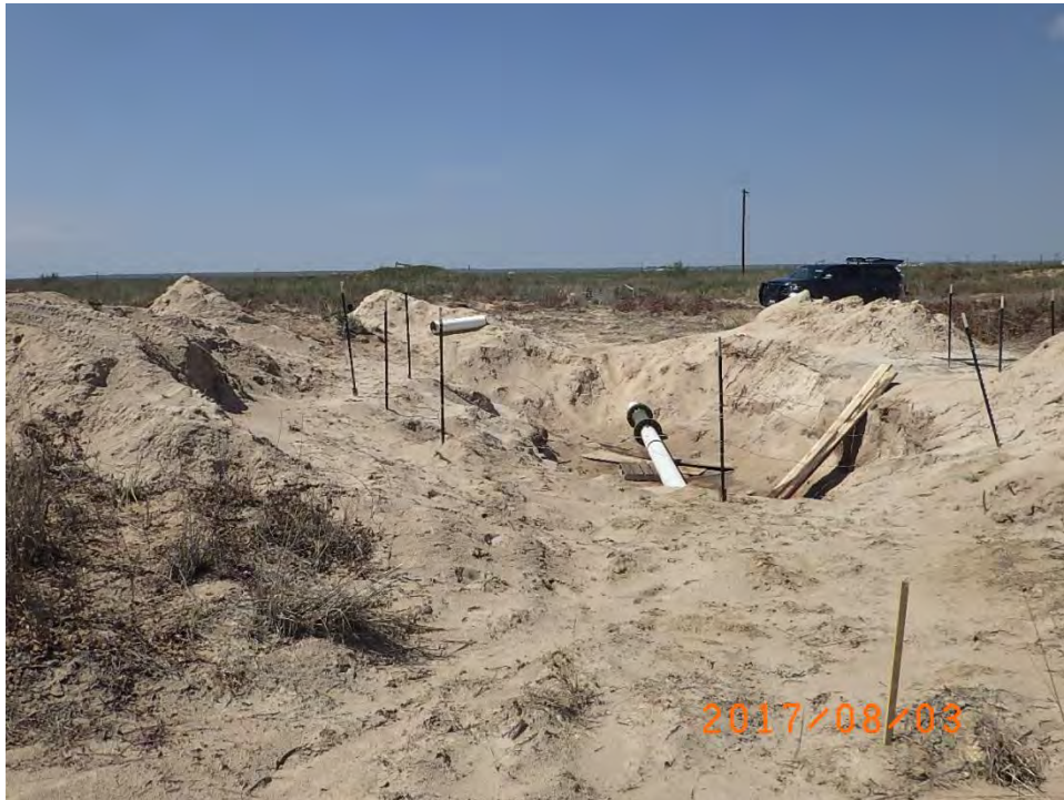
Site Viewing North
