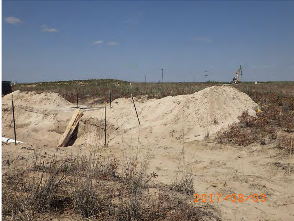
Site Viewing Northeast
