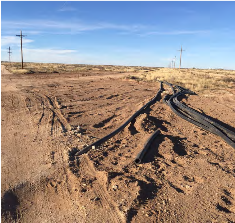
Photo 3 - Backfilled excavation, wheel compacted, re-seeded
