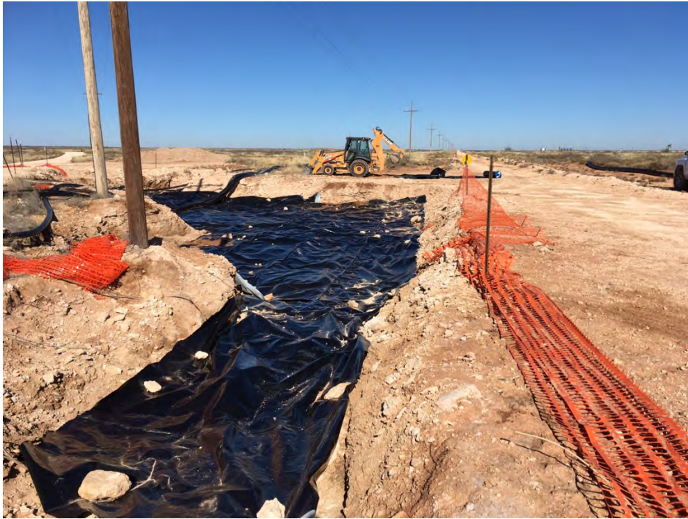
Photo 1 - Liner placement
