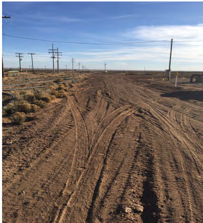
Photo 4 - Backfilled excavation, wheel compacted
