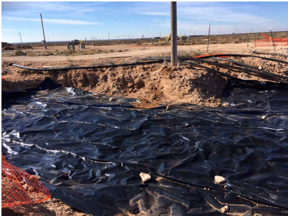
Photo 2 - Liner placement
