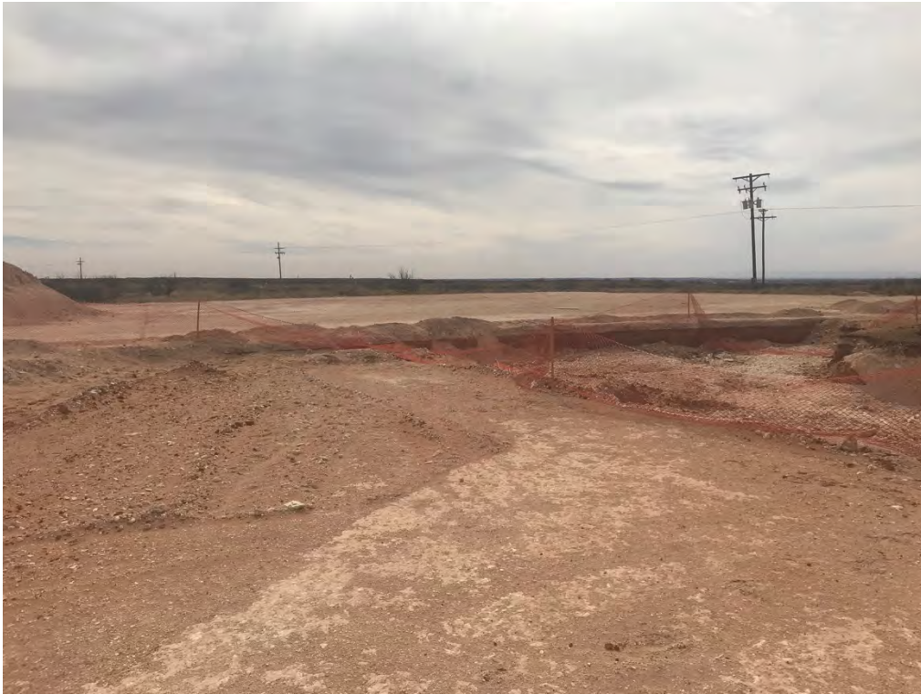
Covington A Federal 0002 – Excavation (Looking South-Southwest)
