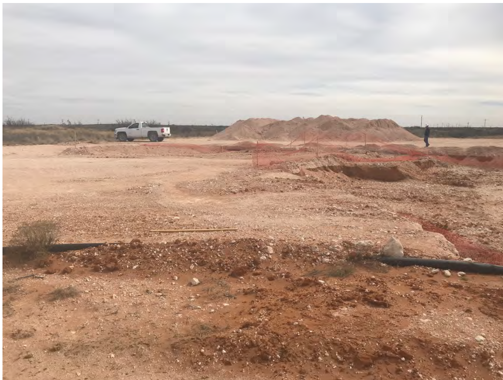
Covington A Federal 0002 – Excavation (Looking Southeast)
