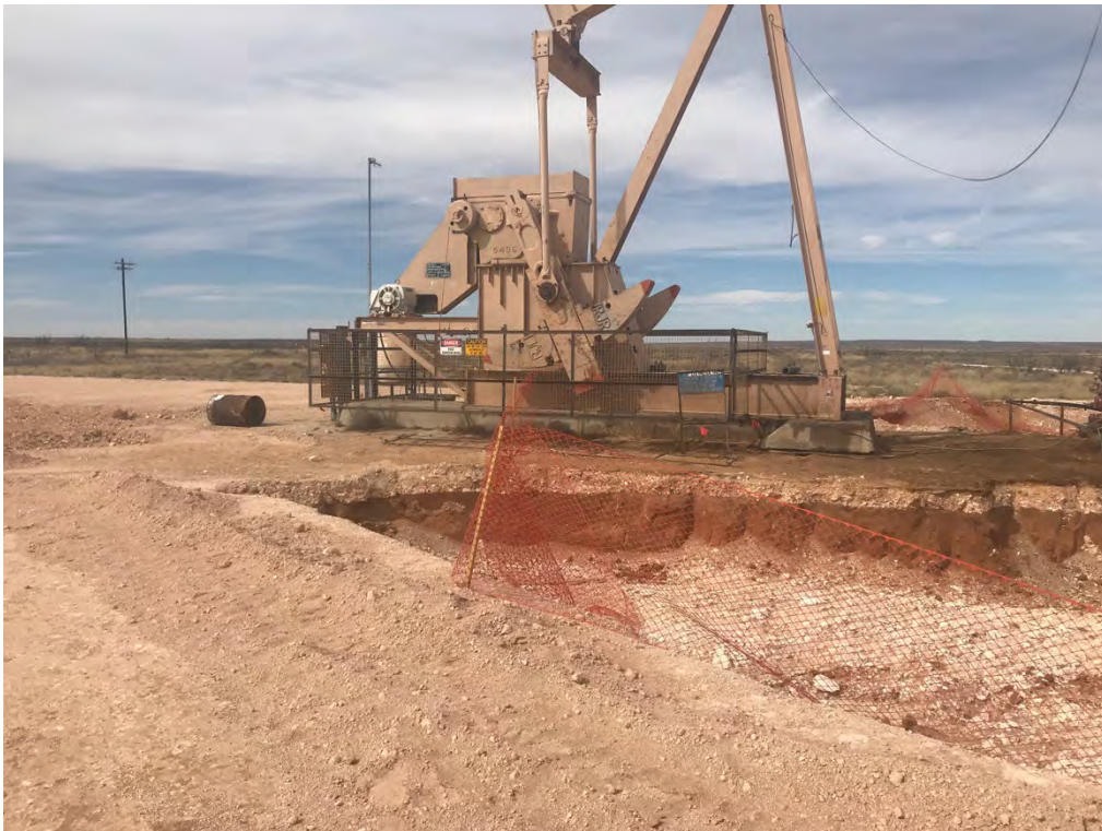
Covington A Federal 0002 – Excavation (Looking North)
