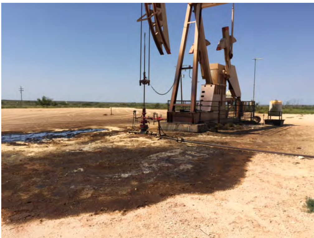
Covington A Federal 0002 – Release (Looking Southwest)
