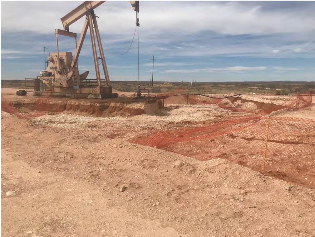
Covington A Federal 0002 – Excavation (Looking Northwest)
