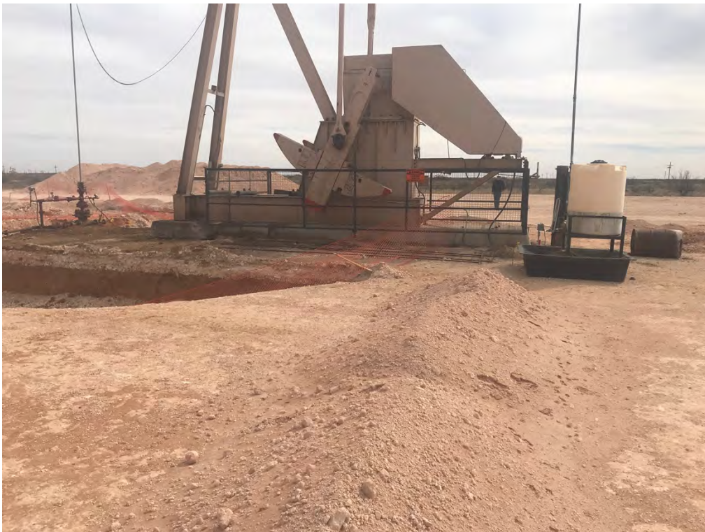
Covington A Federal 0002 – Excavation (Looking South-Southeast)
