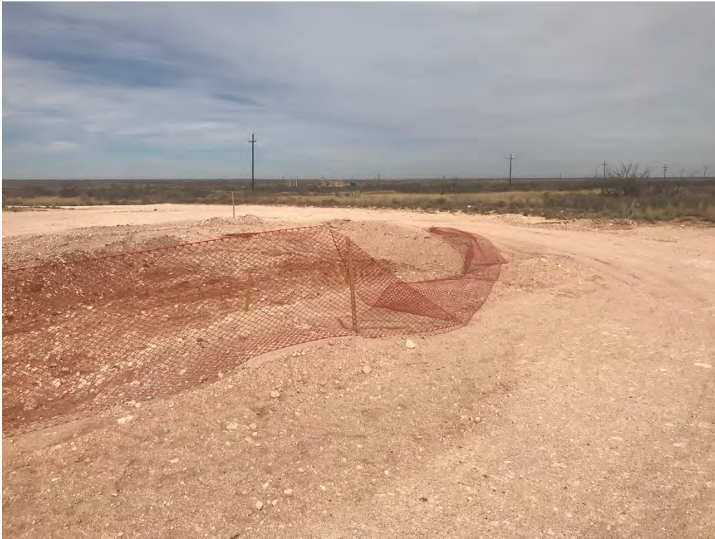
Covington A Federal 0002 – Excavation (Looking East-Northeast)
