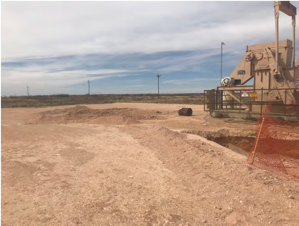
Covington A Federal 0002 – Excavation (Looking North-Northwest)
