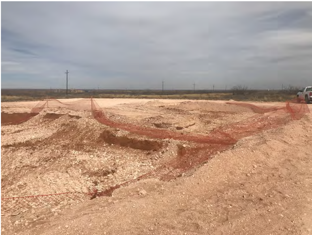
Covington A Federal 0002 – Excavation (Looking Northeast)
