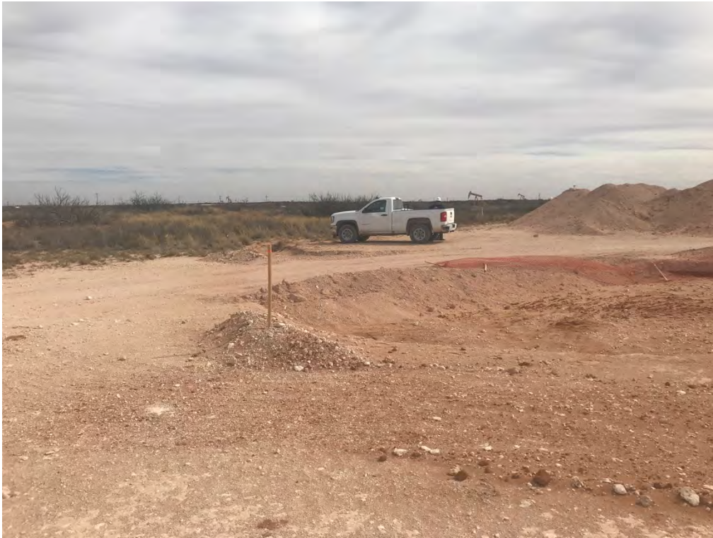
Covington A Federal 0002 – Excavation (Looking Southeast)
