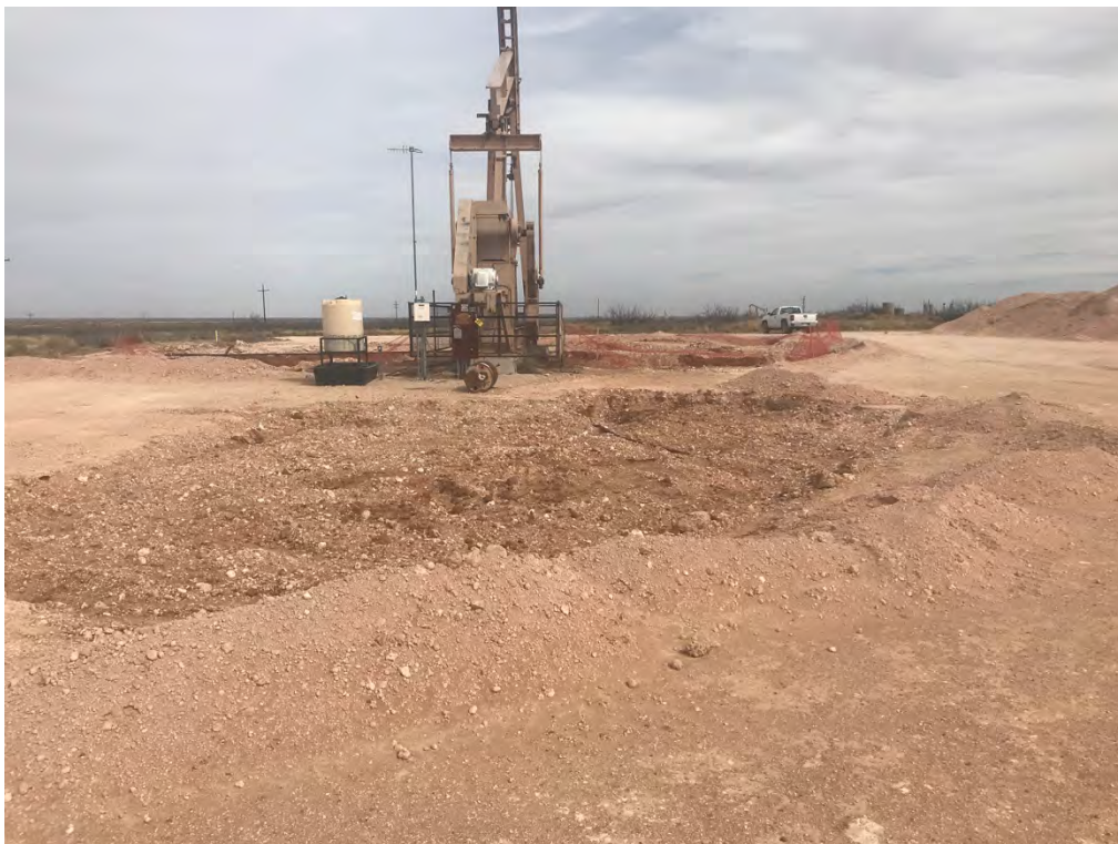
Covington A Federal 0002 – Secondary Excavation (Looking East)
