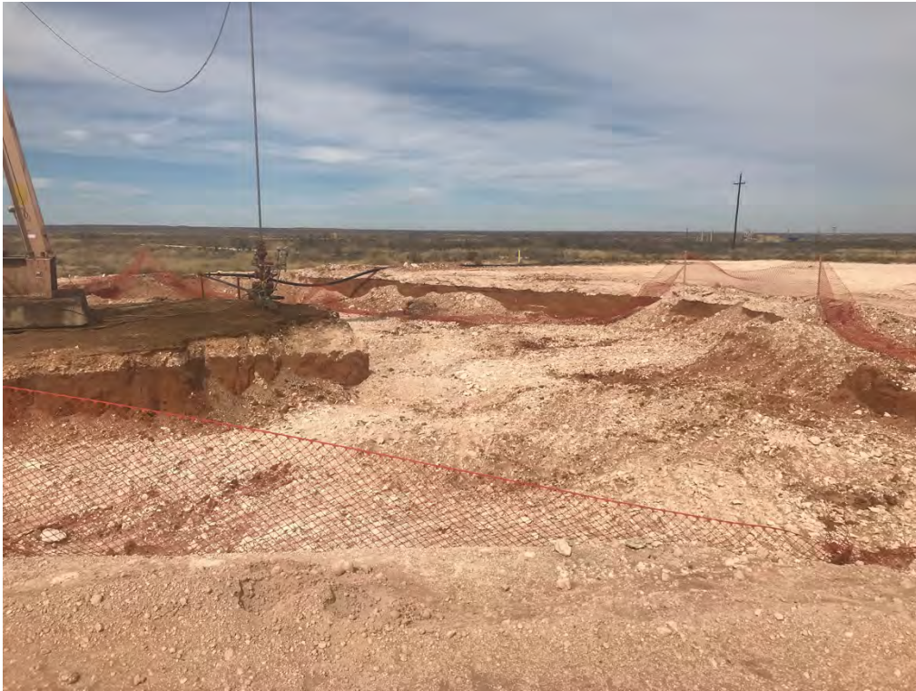
Covington A Federal 0002 – Excavation (Looking North-Northeast)
