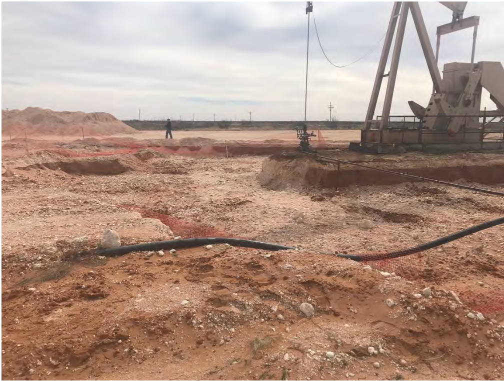
Covington A Federal 0002 – Excavation (Looking South-Southwest)
