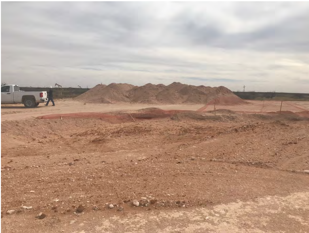
Covington A Federal 0002 – Excavation (Looking Southwest)
