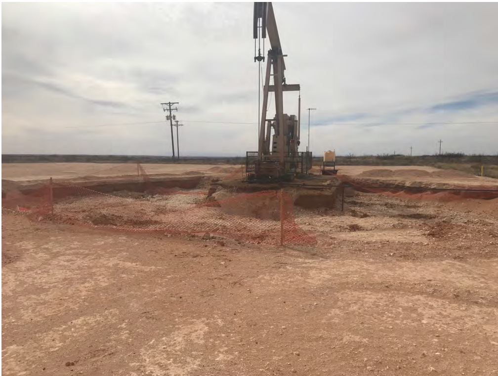
Covington A Federal 0002 – Excavation (Looking West)
