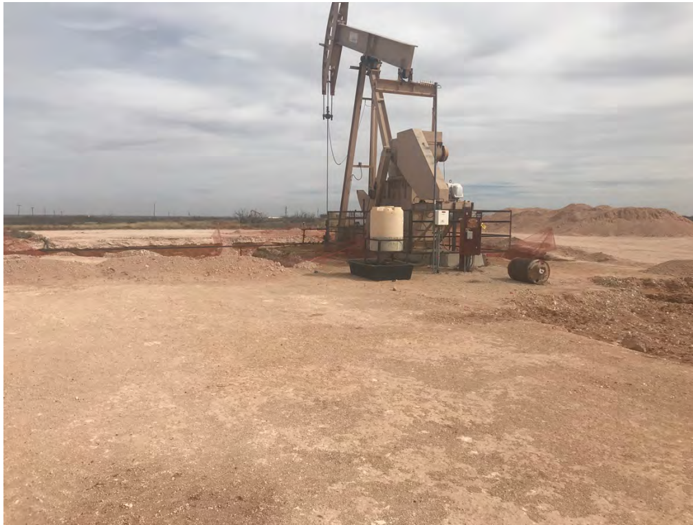
Covington A Federal 0002 – Excavation (Looking East-Southeast)
