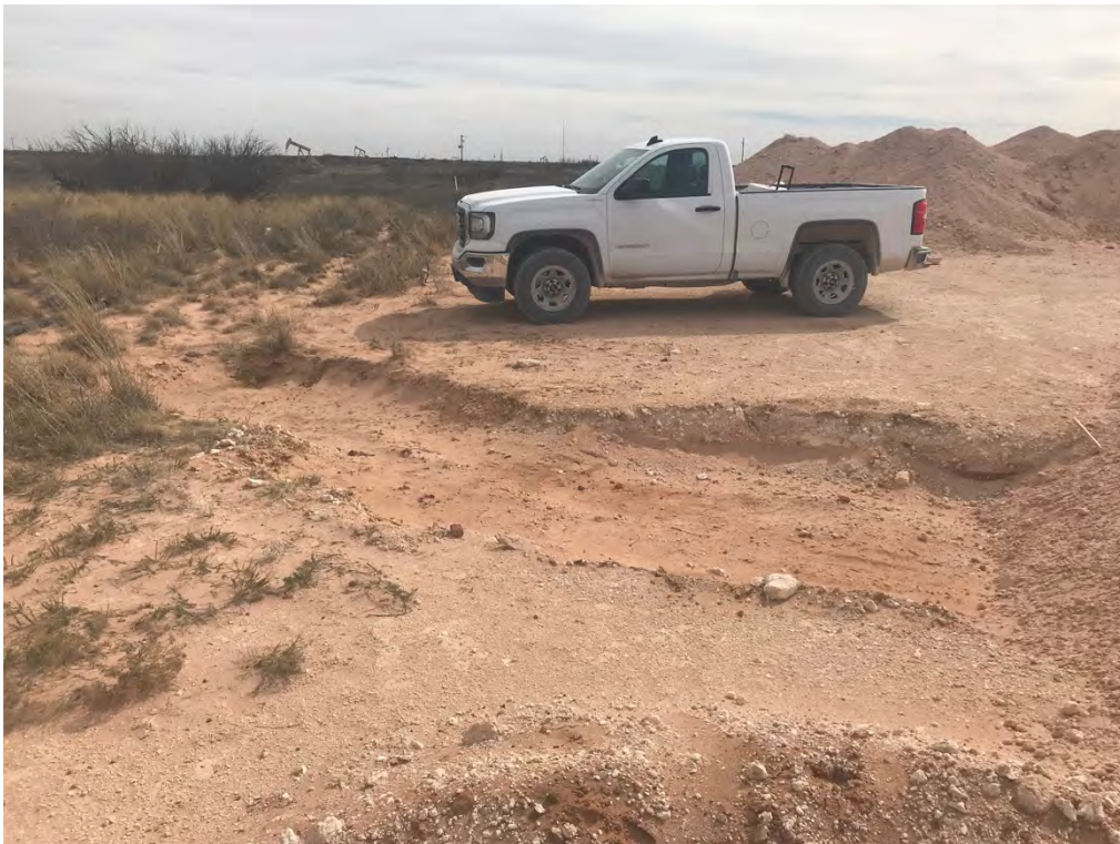
Covington A Federal 0002 – Excavation (Looking South)
