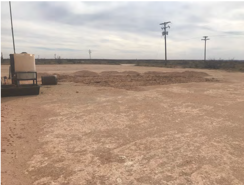
Covington A Federal 0002 – Excavation (Looking South-Southwest)
