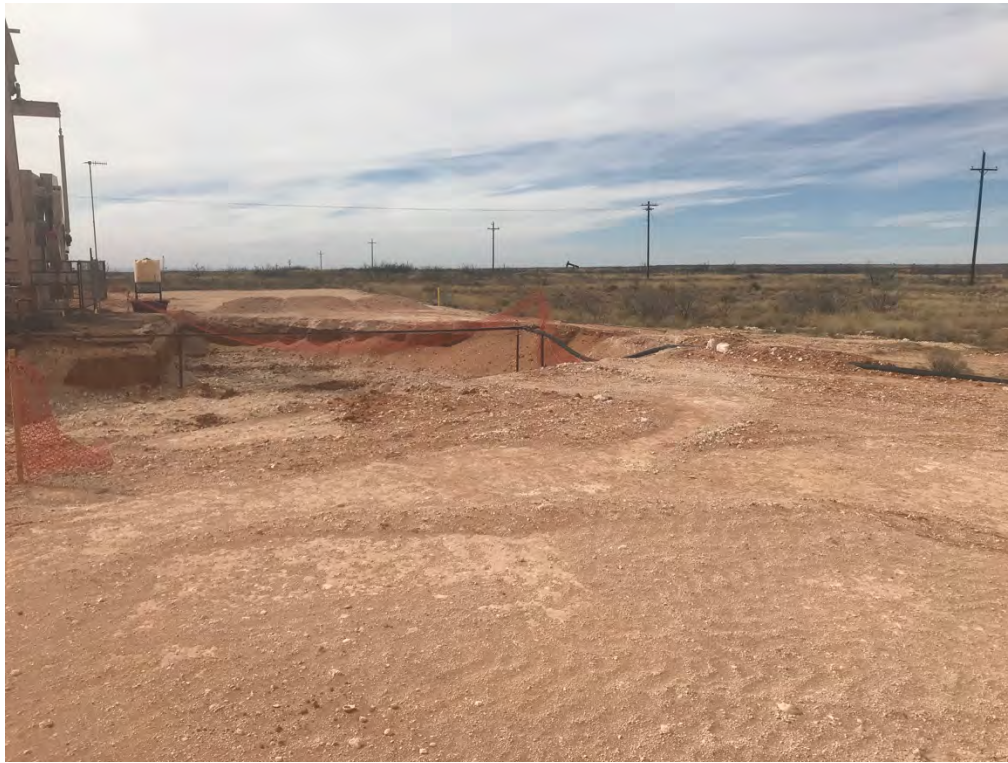
Covington A Federal 0002 – Excavation (Looking West)
