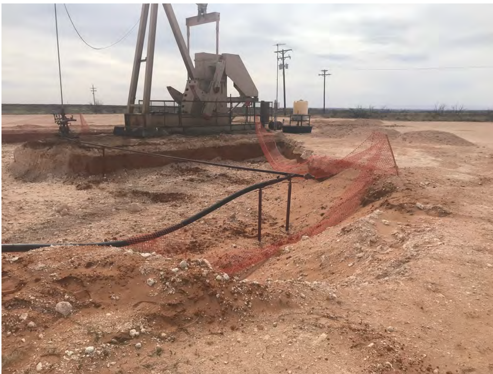
Covington A Federal 0002 – Excavation (Looking Southwest)
