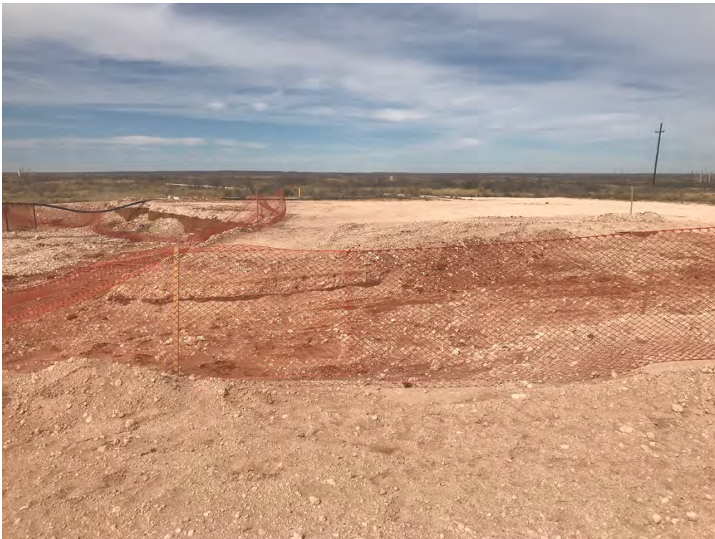
Covington A Federal 0002 – Excavation (Looking North)
