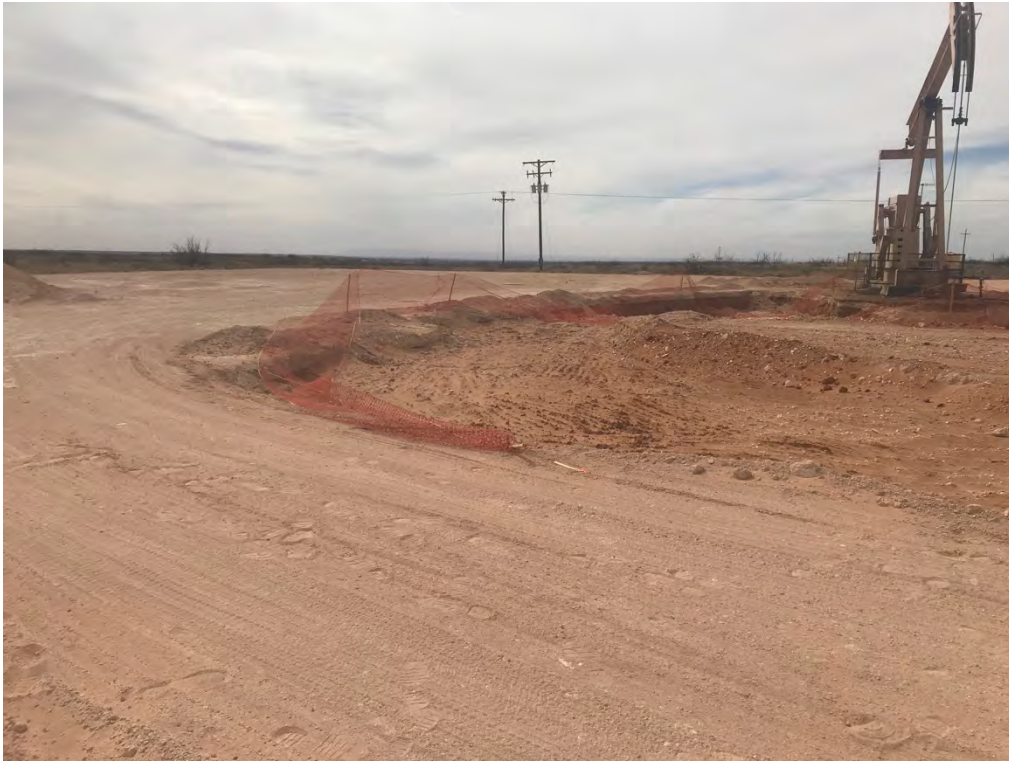
Covington A Federal 0002 – Excavation (Looking West)
