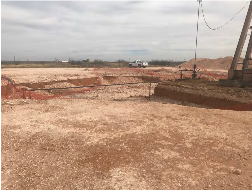
Covington A Federal 0002 – Excavation (Looking Southeast)
