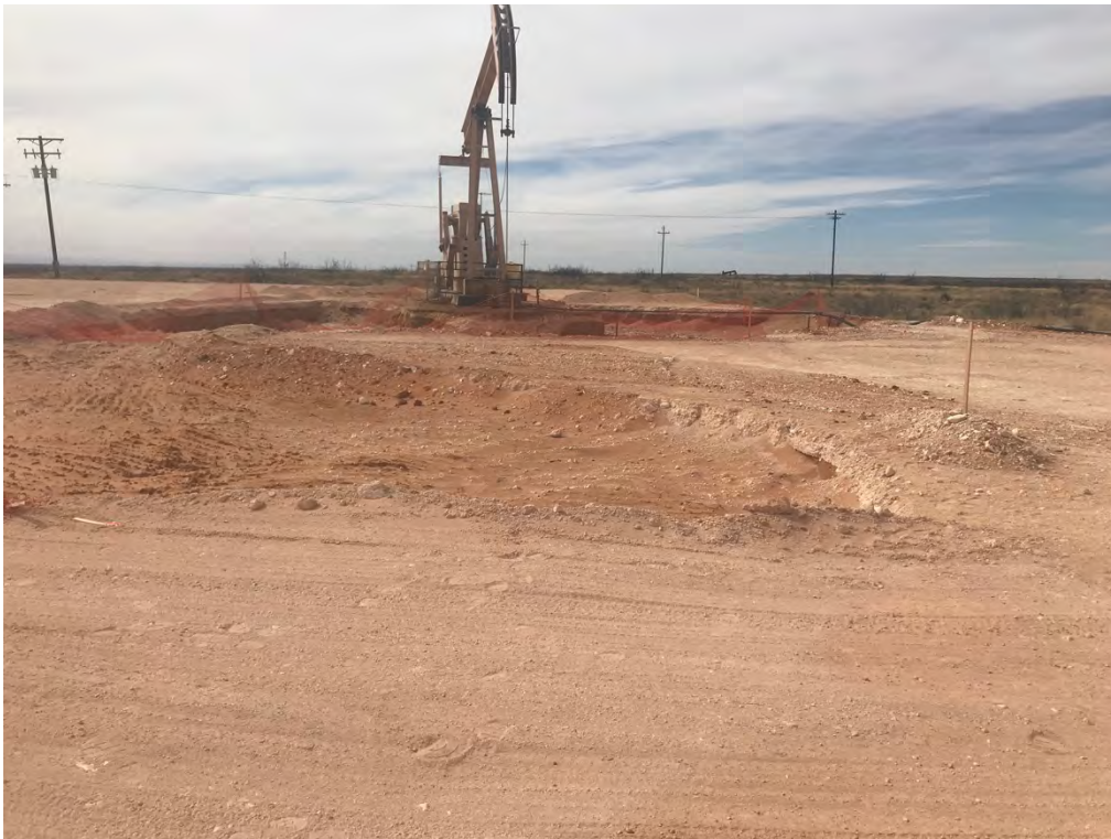
Covington A Federal 0002 – Excavation (Looking West-Northwest)
