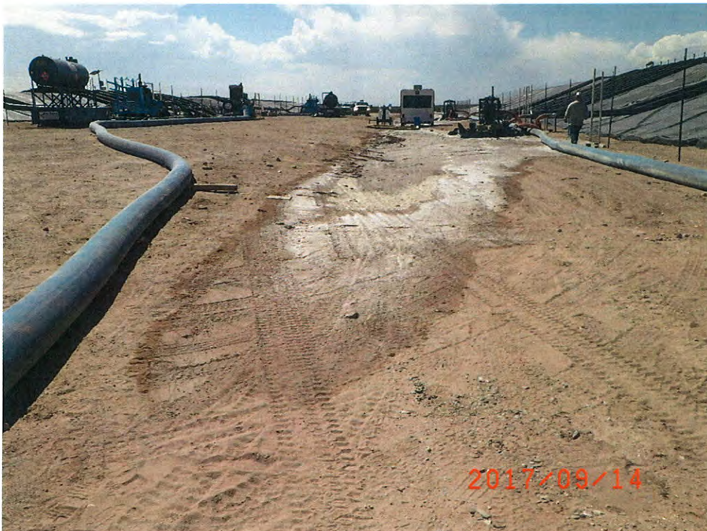
East End of Spill Viewing West
