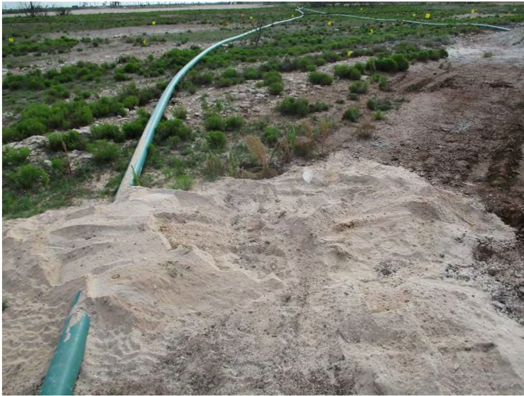
View Northeast - Area of SB-1
